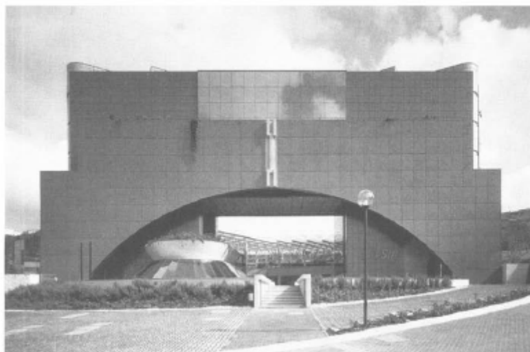
Σχήμα 3.23: The SIP Complex, Ancona, Italy
