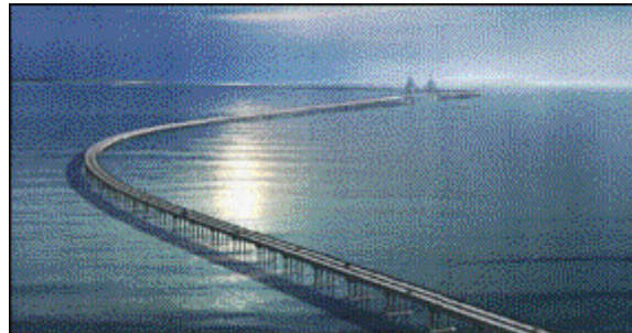
The Donghai bridge
