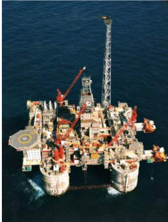
Statoil Heidrun Platform – North Sea Norway (World Largest TLP, First Application of Composite Riser, 1345m)
