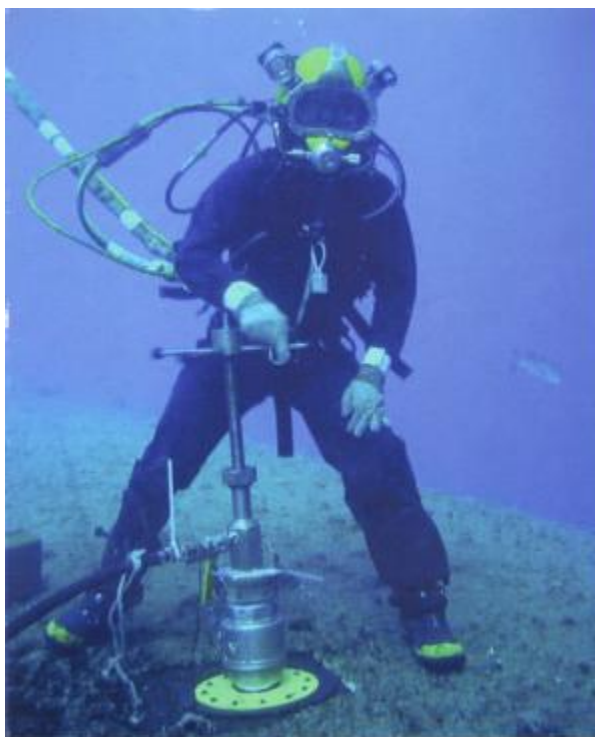
Σχήμα 4.5: Lightweight hot-tap.
