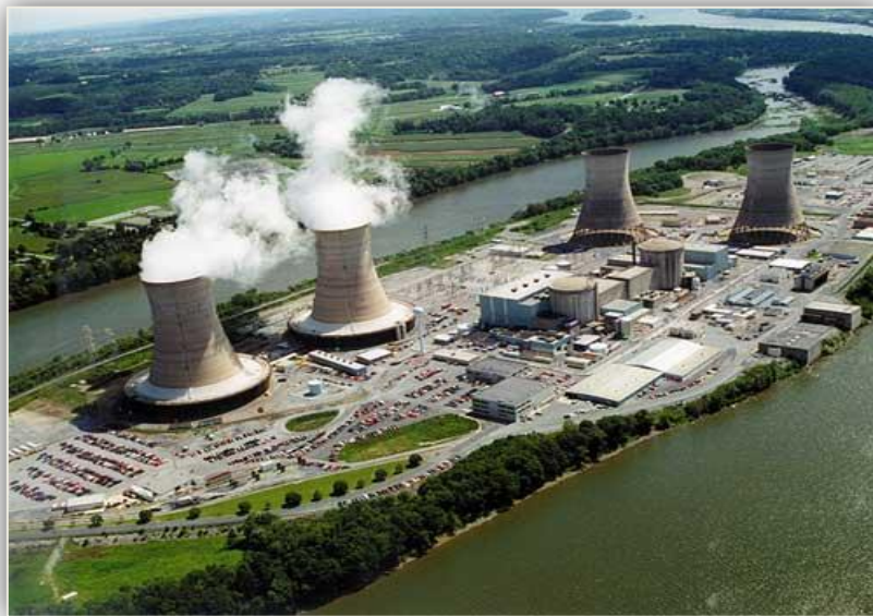
Figure 3. 13: Three Mile Island nuclear power plant
