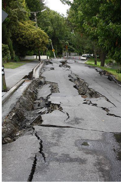
Figure 1.4: Soil liquefaction occurred after the earthquake in Christchurch in 2011
