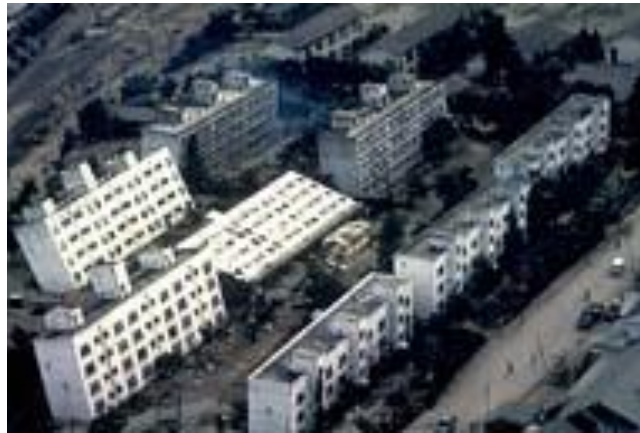
Figure 3.4.3: Buildings sloping during the 1964 Niigata earthquake
