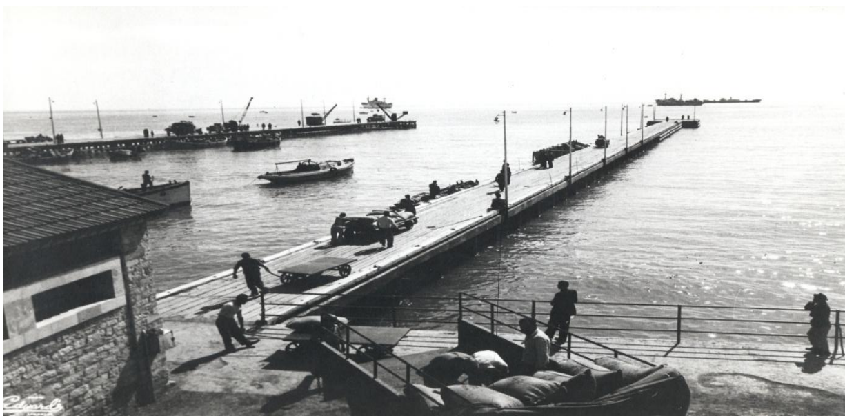
CONCRETE JETTY, OLD HARBOUR, LIMASSOL, CYPRUS 1954
