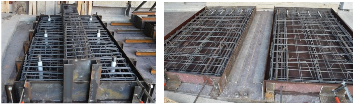
Figure 8.6. Photos of the specimens after placement of the reinforcement.
