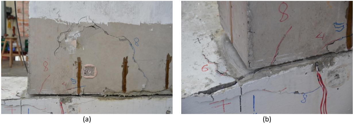
Figure A.19. Test A1D25C-G: Damage observed at the end of the test: (a) spalling of the concrete around the rebar in the area of the joint; (b) spalling of the concrete of the beam.
