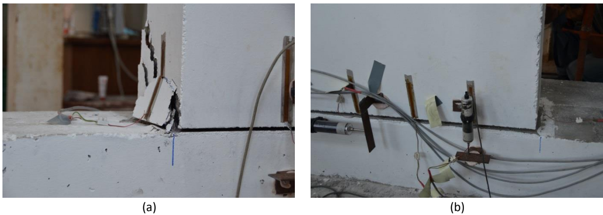
Figure 9.10. Test A1D20C-R1: Damage observed at the end of the test: (a) spalling of the concrete on the left side; (b) no evident damage on the right connection.
