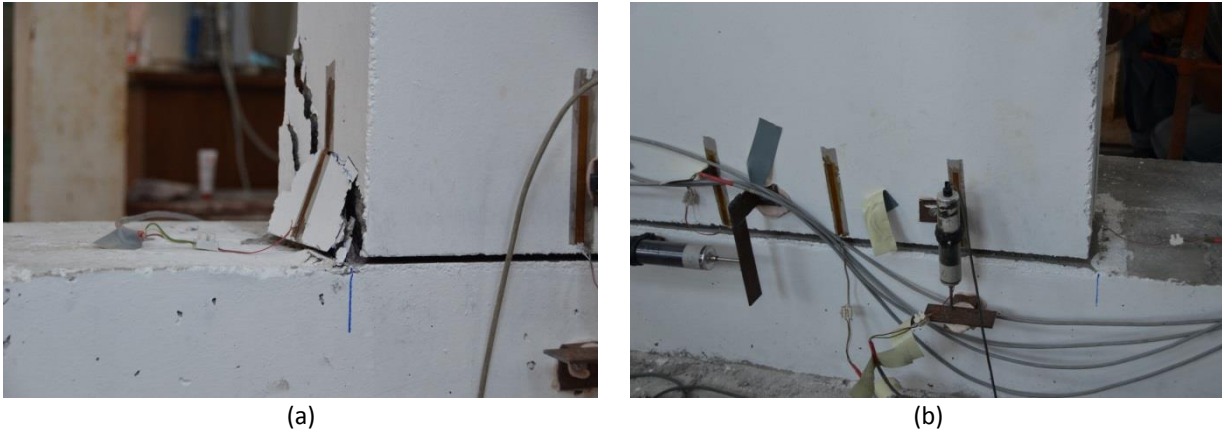
Figure A.7. Test A1D20C-R1: Damage observed at the end of the test: (a) spalling of the concrete on the left side; (b) no evident damage on the right connection.
