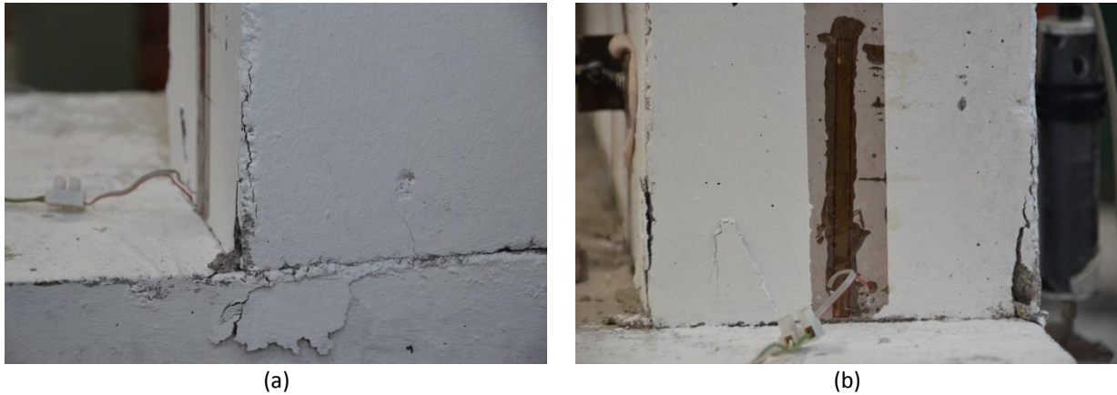
Figure A.15. Test A1D25M-G: Spalling of the concrete of the panel and the beam on the compression side at the end of the initial monotonic loading.
