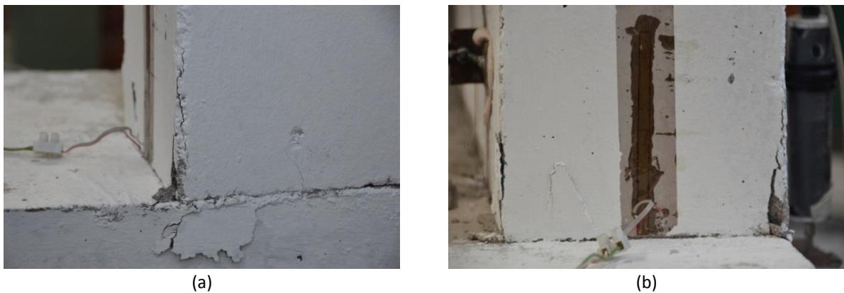
Figure 9.18. Test A1D25M-G: Spalling of the concrete of the panel and the beam on the compression side at the end of the initial monotonic loading.
