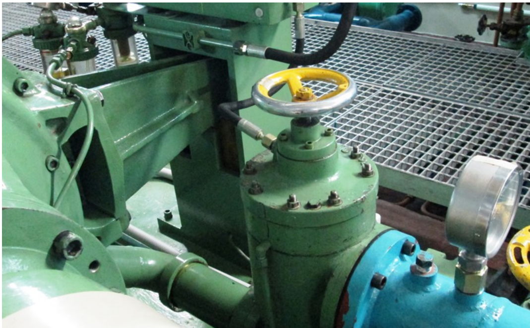
Figure 3.20: Water output analog valve and arm with loadcell
