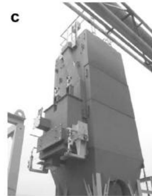
Equipment for cleaning off-gases containing solid particulates, \text{SO}_2 , HCl, HF and heavy metals and alternatively \text{NO}_x , or PCDD/F
