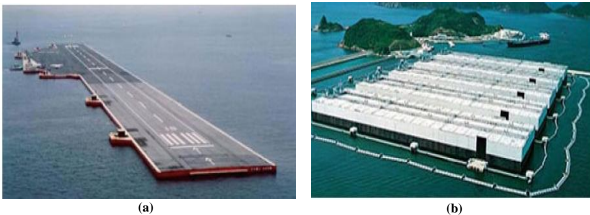
Figure 3 Pontoon type VLFS applications (a) Mega-Float-Tokyo Bay (b) floating oil storage base -Kamigoto island (source: [11])
