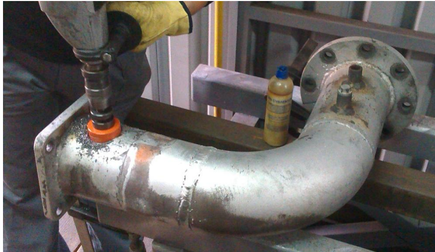
Figure 3.4.3. Drilling holes on the exhaust duct.
