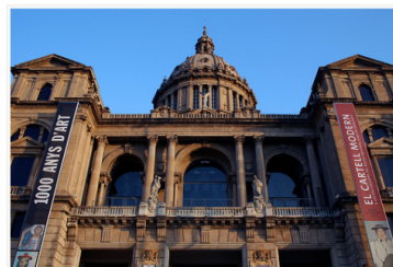
Suggested tags: Montjuïc circuit, Museu Nacional d'Art de Catalunya, Barcelona Frequent user tags: Montjuïc, castellers, Travelling Pooh, architecture, mnac
