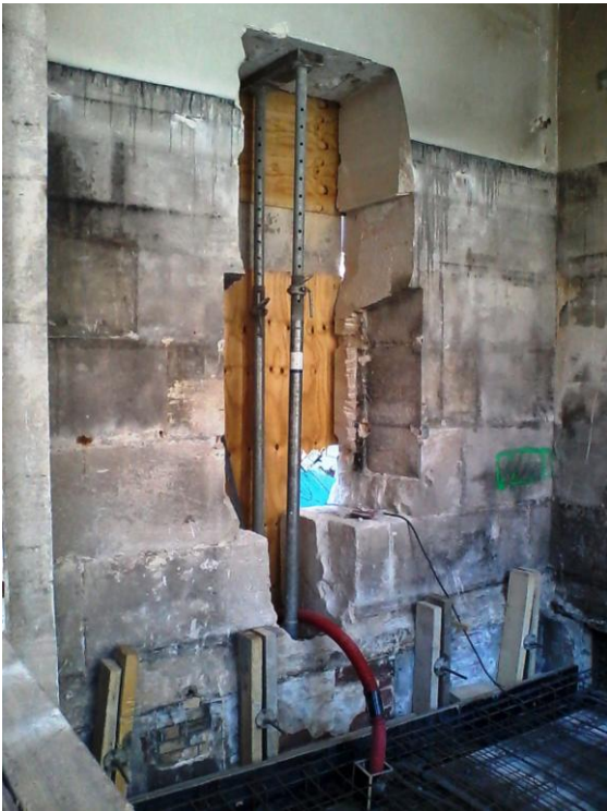
Figure 117 Etais supportant l'ouverture
