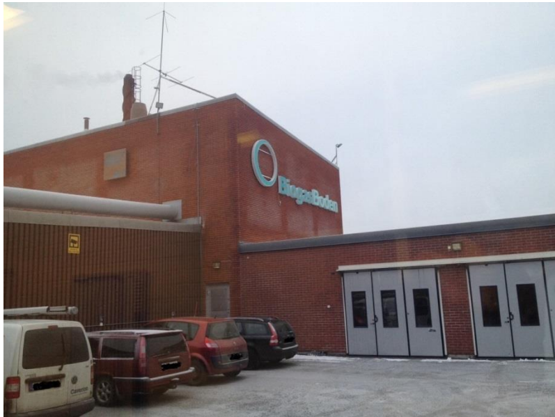
Figure 12: The biogas plant in Boden, Sweden, source of the thermophilic sludge.
