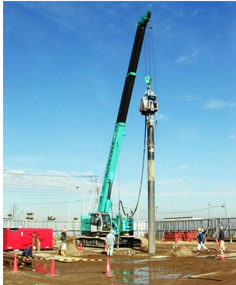
Figure 3.46: Vibratory pile used for shaking induced liquefaction.
