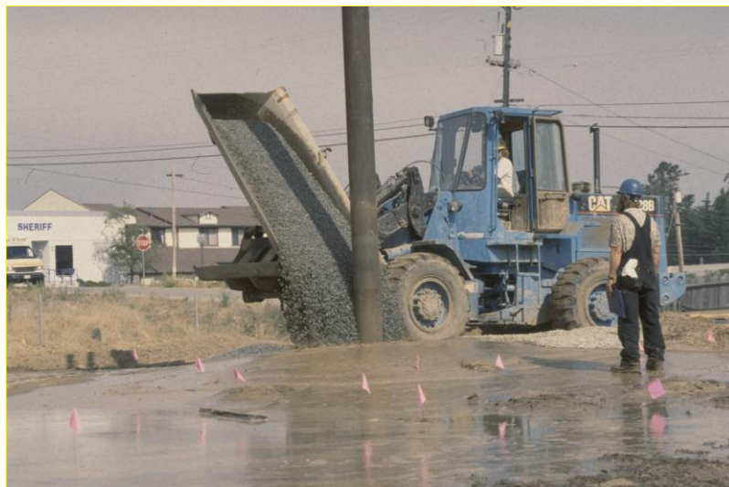
Figure 2.5: Snap-shot of the wet top feed method (Nilex Inc.).
