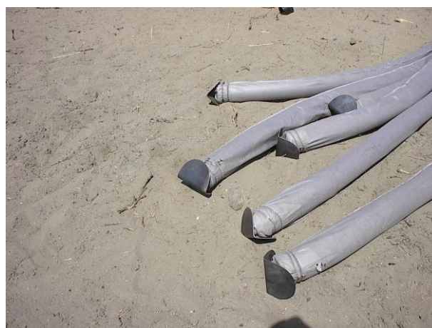
Figure 3.6: Pre-assembled EQ-drains with the specially configured anchorplate (Nilex corporation).
