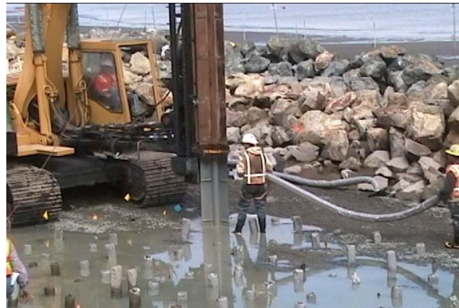
Figure 3.5: Installing EQ-drains at a construction site (Bay bridge project Nilex Corporation).
