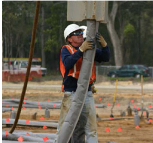
Figure 3.4: Feeding the EQ-drain into the mandrel (Ellington Cross LLC).
