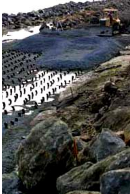
Figure 3.8: EQ-drains installed and reservoir under construction (Bay bridge project Nilex, Corporation).
