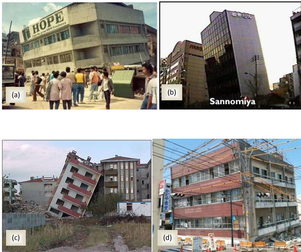
Figure 1.1: Liquefaction-induced failure of shallow foundations from various earthquakes (a) Dagupan, Philippines, 1990, M=7.8 , (b) Kobe, Japan, 1995, M=7.2 (c) Adapazari, Turkey (1999) M=7.4 , (d) Sendai, Japan, 2011 M=8.9 .
