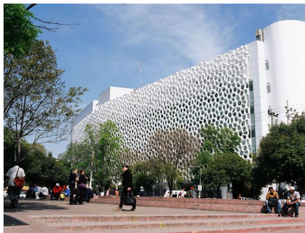
Fig. 1. Hospital in Mexico City; building façade with self cleaning properties, year 2011 [2]
