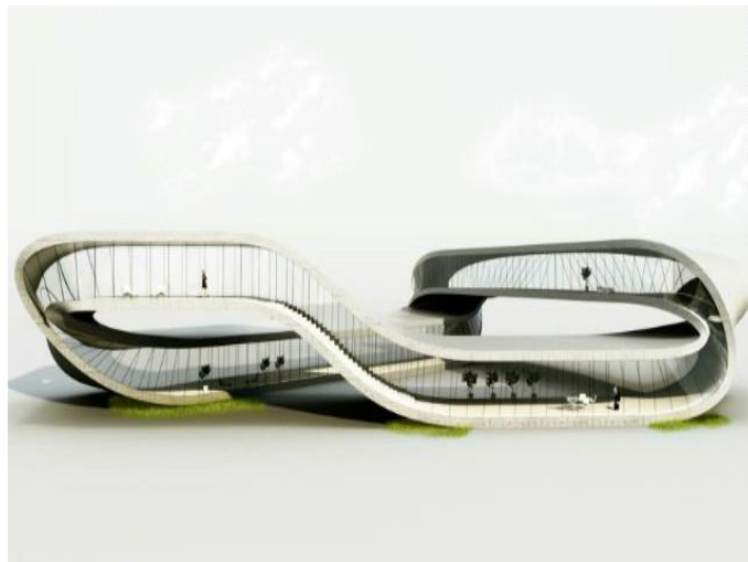
Fig. 8. Landscape House, Amsterdam. This ia a Möbius strip-shaped building ‘printed’ all in one go with one huge 3-D printer created by Italian roboticist E. Dini, arch. J. Ruijssenaars [35]
