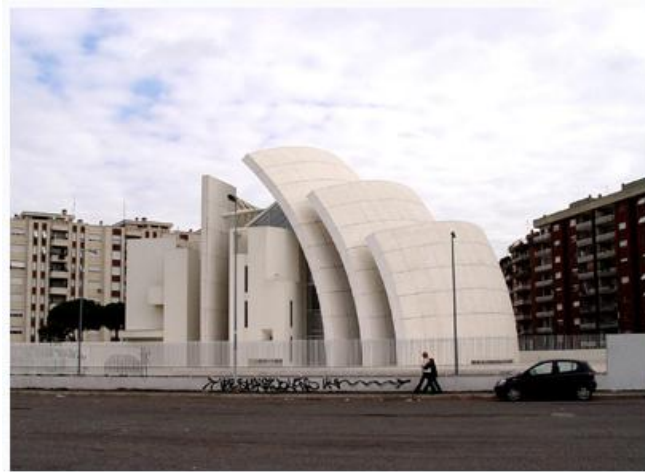
Fig. 2. Misericordia church in Rome made of exposed white concrete with self cleaning properties, year 2003, arch. R. Meier & partners [5]
