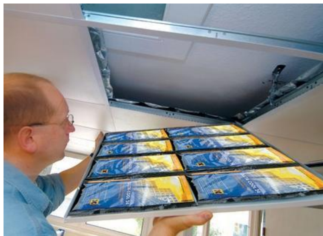
Fig. 5. Phase change materials for thermal energy storage, built in a room’s ceiling [11]
