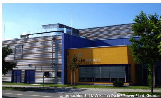
Figure 20: The Unterhaching Kalina Power Plant ( www.geothermie-unterhaching.de )
