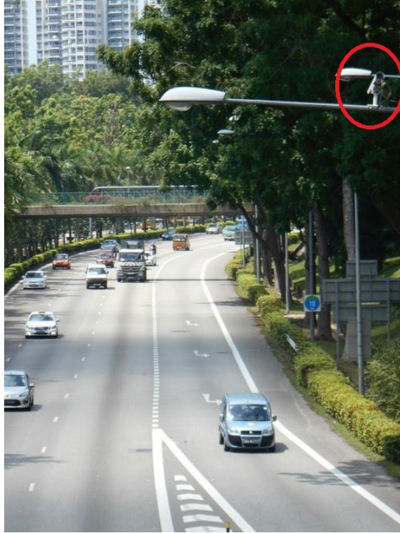
Figure 5.2: Example of cameras that measures traffic flow on Singapore expressways (photo taken by Stephen Robinson)
