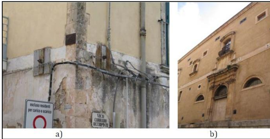
Figure 4.8: the application of horizontal tie rods on masonry walls (Rashadul 2008)
