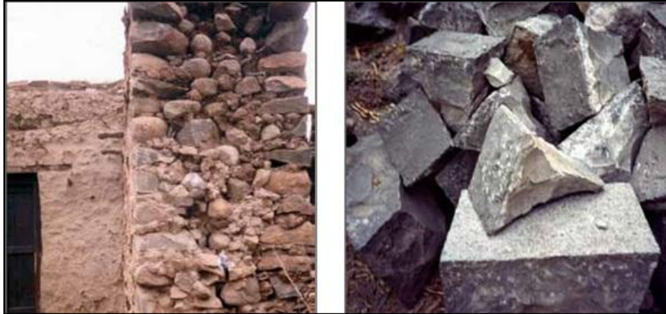
Figure 1.52 Round stone boulders used for traditional stone masonry and semi-dressed stones ready for wall construction (Bothara and Brzev 2011)
