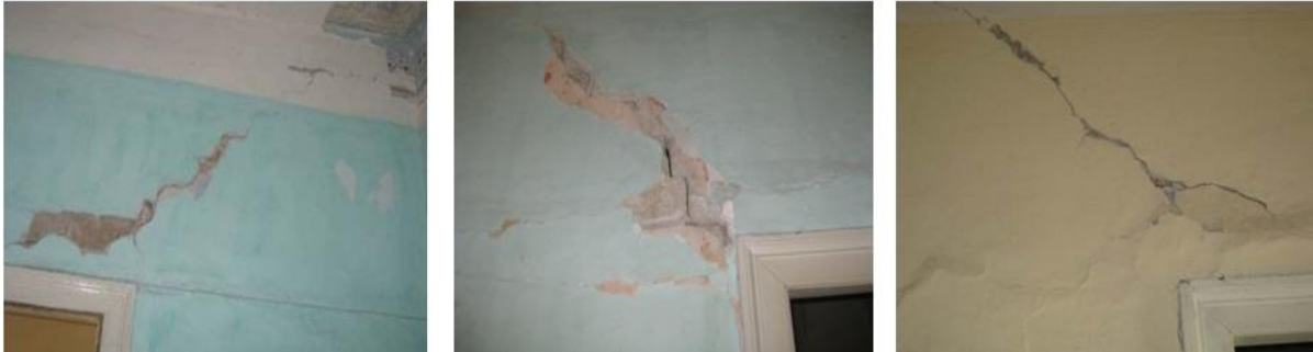
Figure 5.43: Typical diagonal cracking of secondary wall
