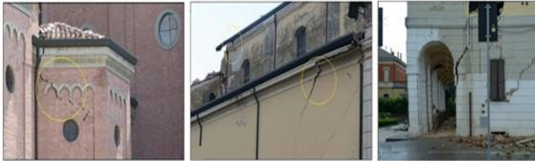
Figure 2.35 Cracks aspects in historic traditional masonry buildings in Italy (Pauperio E. et al 2012)
