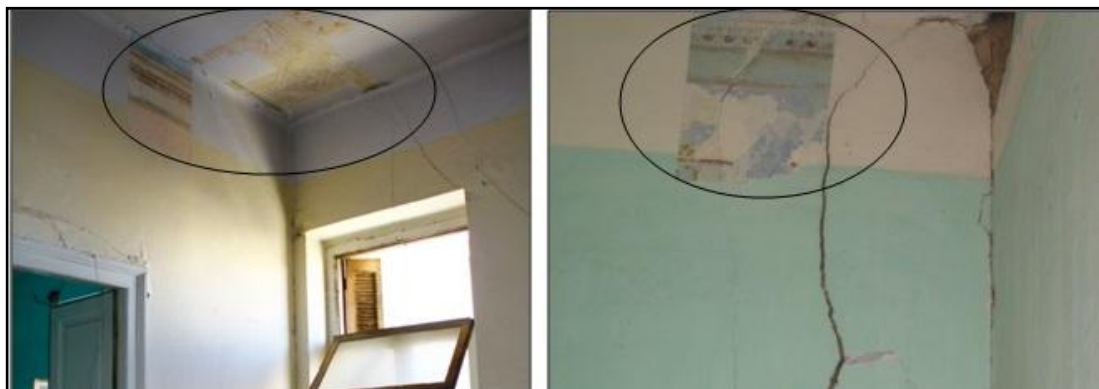
Figure 5.9: shows over painting covering original wall paintings
