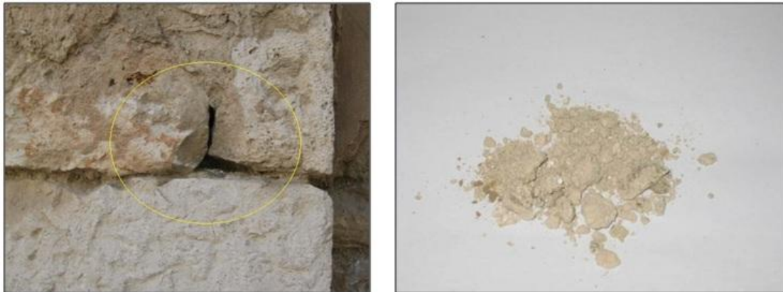
Figure 5.52: Fragmented mortar
