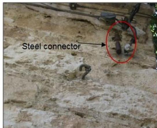
Figure 5.18: Steel connector tying orthogonal walls and roof
