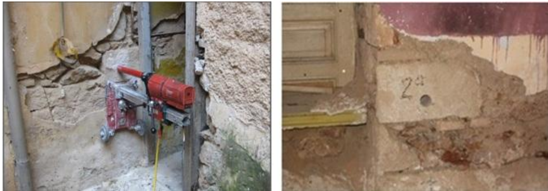
Figure 5.60: Drilling core from a ground floor stone
