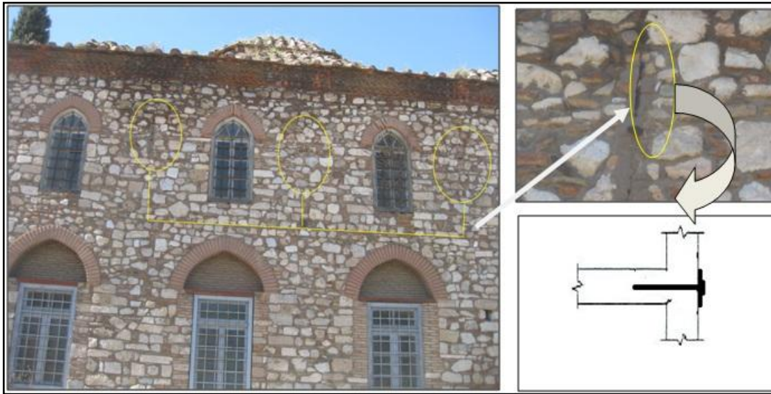
Figure1.28 Positioning of three steel ties in historic traditional building ( Alfatihia Mosque)
