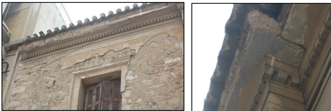
Figure 5.39: Wall cracking at the top of the building (W2-ex, 1 st floor)
