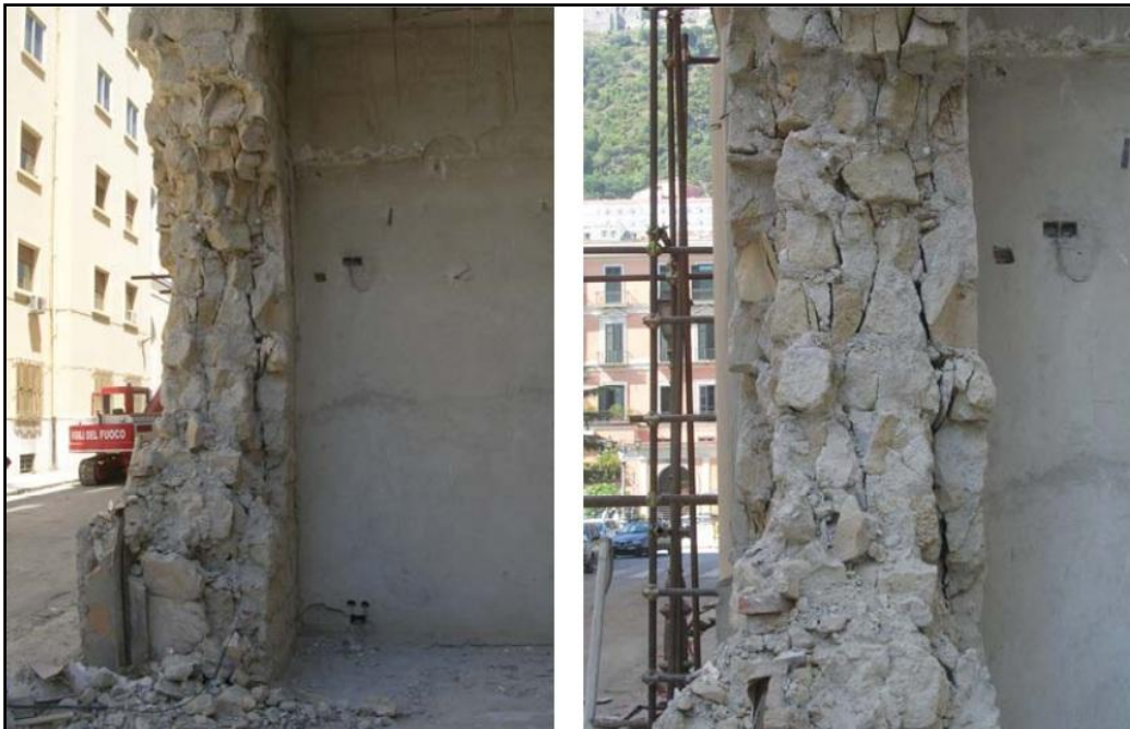
Figure 2.32 The use of poor building materials and poor mortar bond (Augenti, N. 2008)
