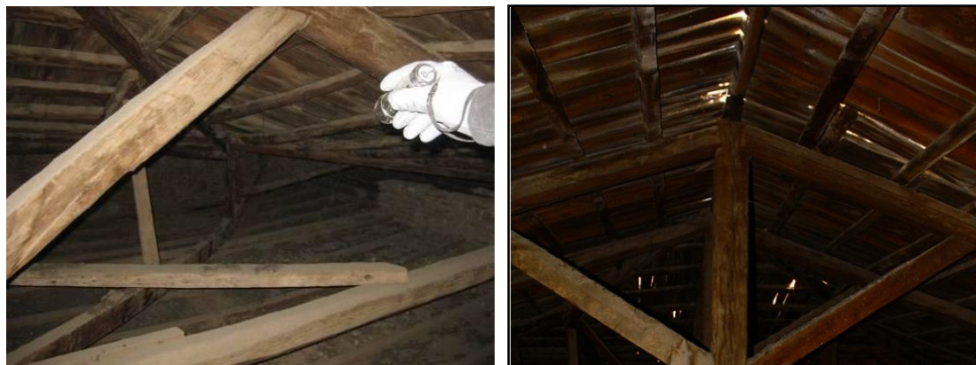
Figure 5.46: Excessive truss deflection
