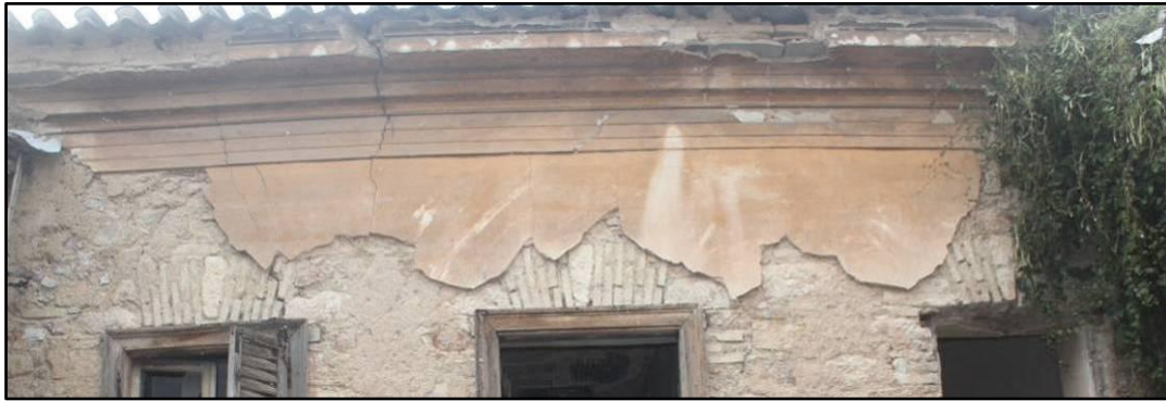
Figure 5.36: Typical lintel of external opening
