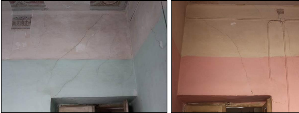
Figure 5.71: Masonry cracking supported by door wooden lintel
