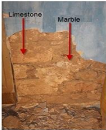
Figure 5.16: Wall masonry
