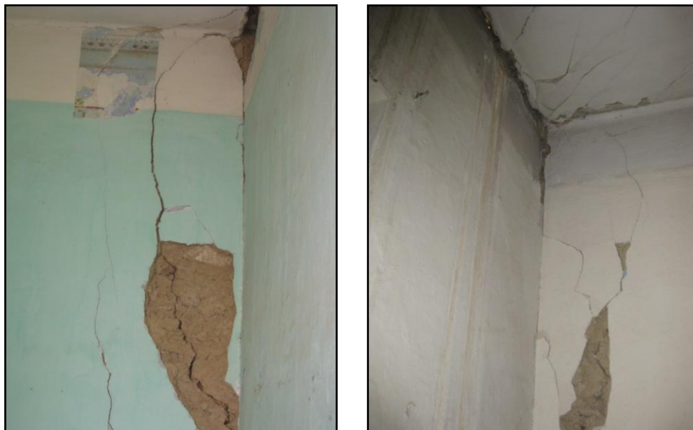
Figure 5.69: Near vertical near the primary wall intersection
