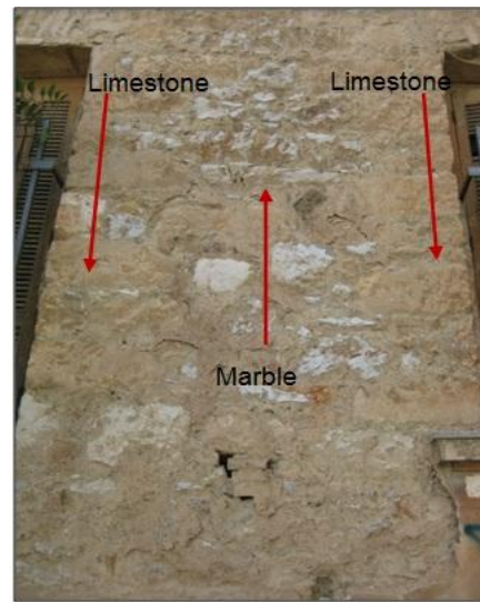
Figure 5.17: Wall and window cornerstones
