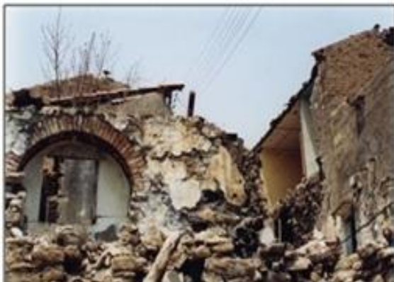
Figure 2.5 Total collapse of construction
