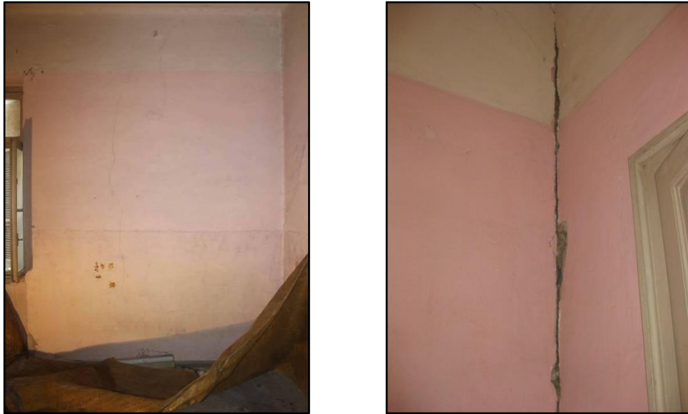
Figure 5.73: Detachment of non bearing walls from bearing walls at 1 st level due to lack of connection
