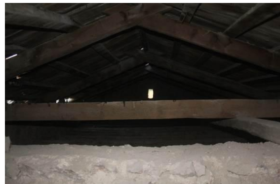
Figure 5.28: Truss of wing roof
