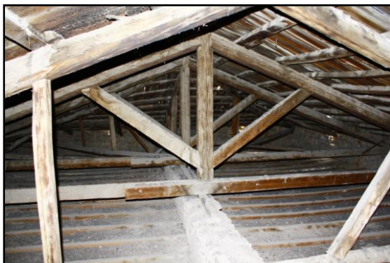
Figure 5.27: Truss of central roof
