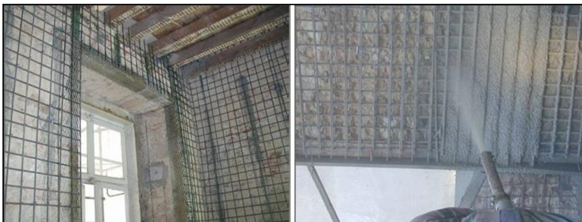
Figure 5.81: Steel mesh of cement paste coating
