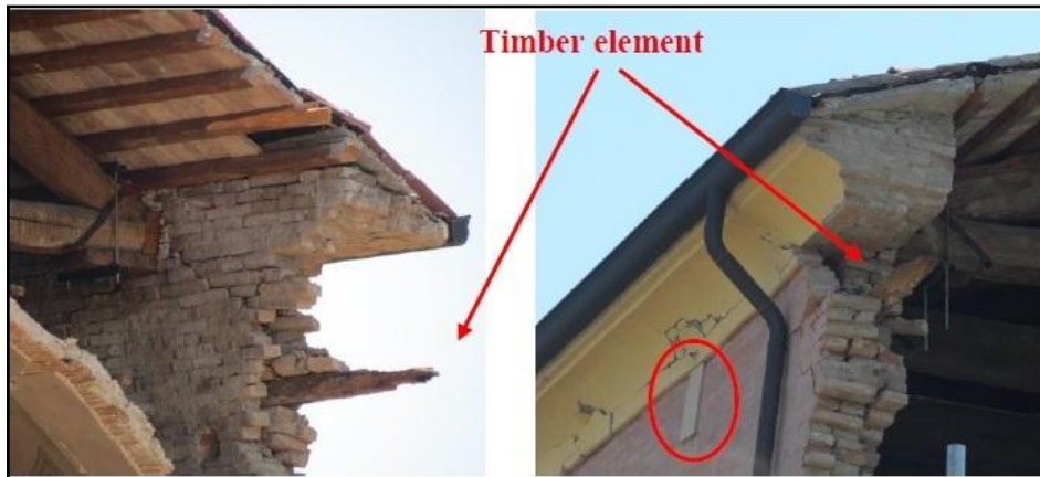
Figure 1.21 Timber elements inside the brick walls
