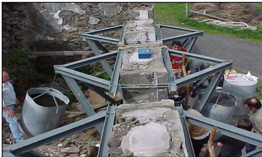
Figure 3.19 - General view of the experimental set-up used to perform the tests (after Costa and Arede 2006)
