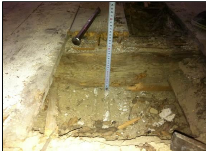
Figure 5.22: Spacing of beams of ground level floor
