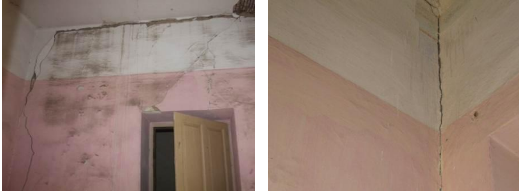
Figure 5.41: Vertical crack near wall connection (W6-in, 1 st floor)
