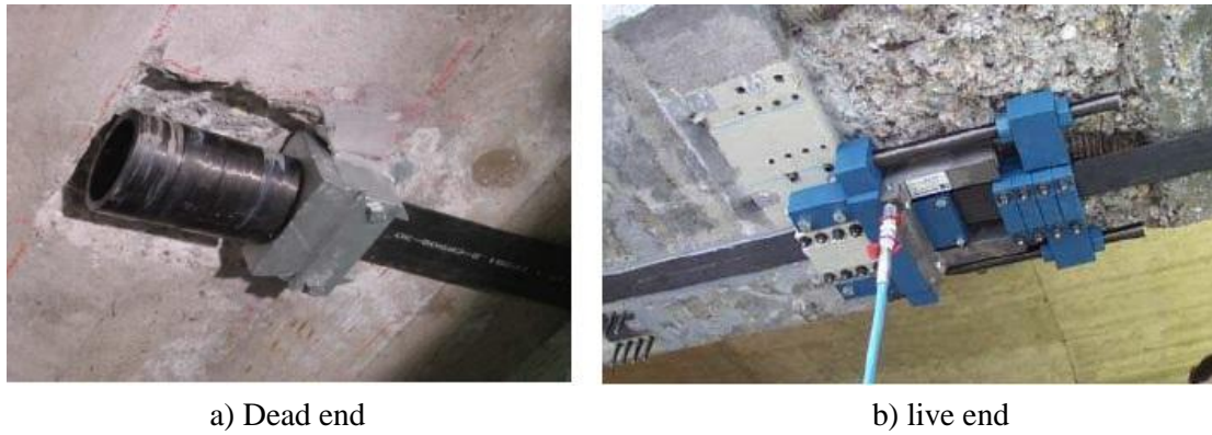
Figure 4.12 Applying Post-Tension (Rashadul 2008)
