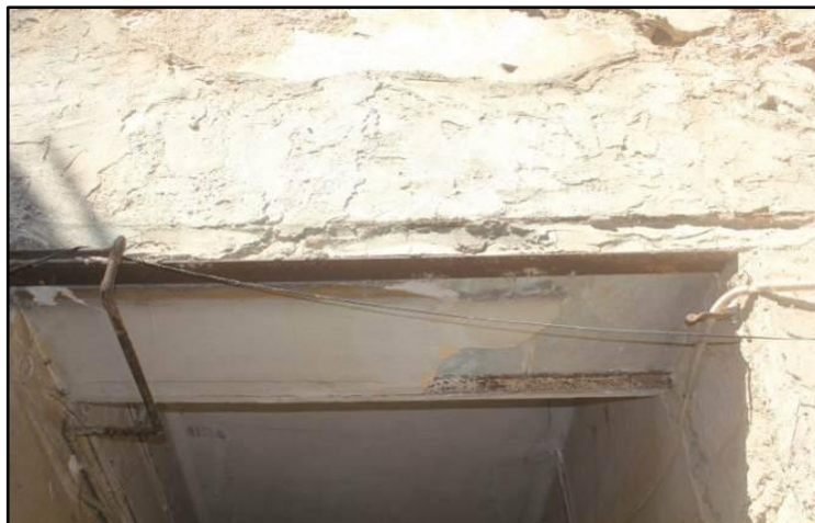
Figure 5.37: Metal support of door lintel
