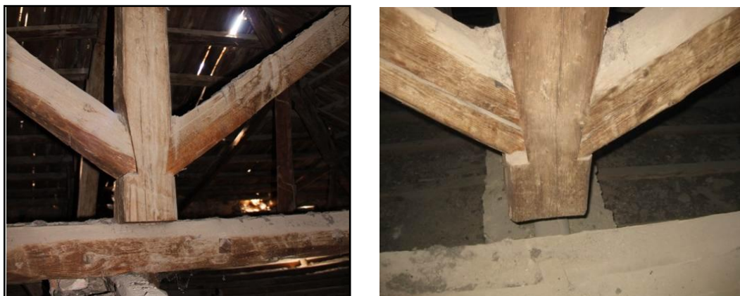
Figure 5.44: Truss deviation from vertical
