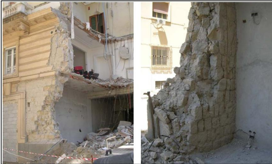
Figure 2.31 Partial collapse in Salerno building (Augenti, N. 2008)
