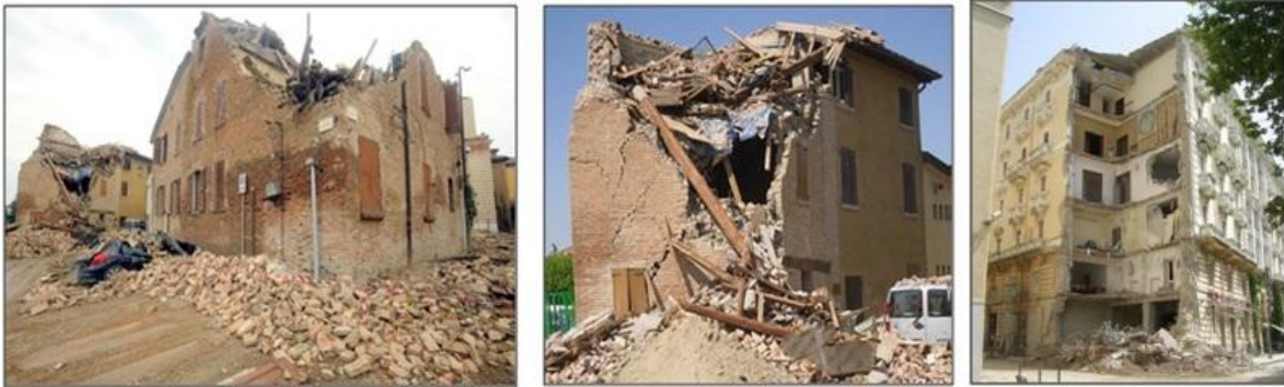
Figure 2.8 Out-of-plane corner mechanisms of masonry building units located in the historical center of San Felice sul Panaro and Salerno building (Branco M., 2011, Augenti, N. 2007)
