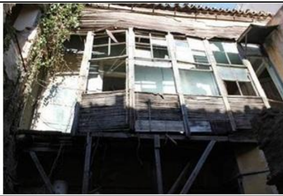
Figure 5.33: Typical gallery looking in the internal open space with temporary prop
