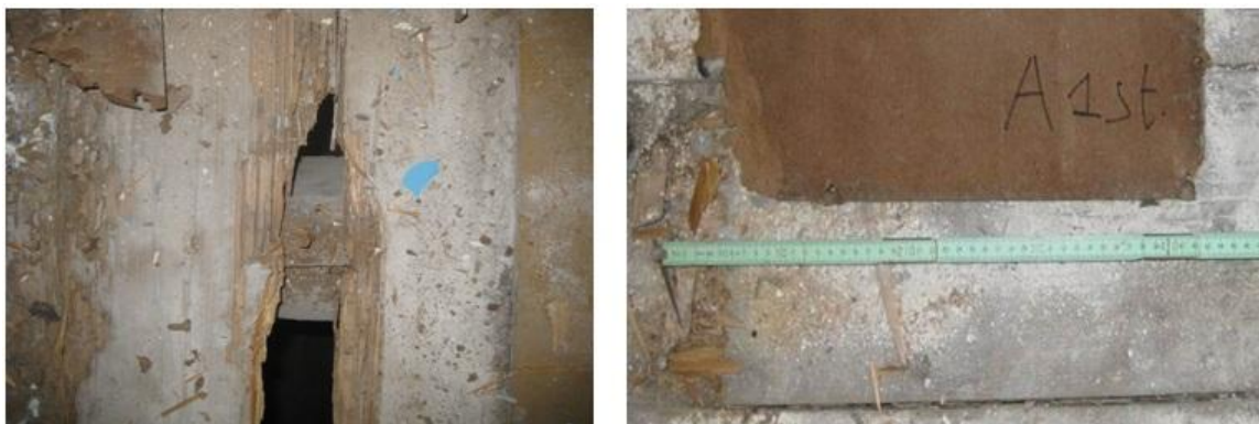
Figure 5.24: Spacing of beams of 1 st storey floor
