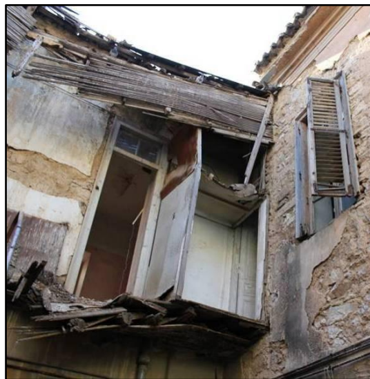
Figure 5.34: Typical gallery in a state of collapse.
