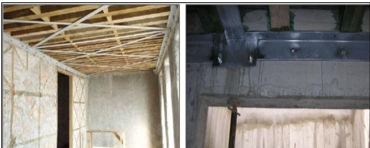
Figure 4.14 In plan stiffening with metallic diagonal and L shaped steel plates as connection reinforcement between walls and floor.
