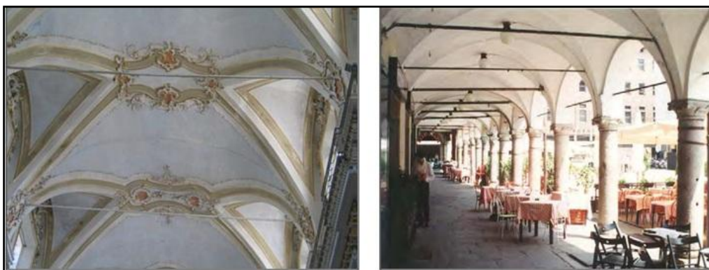
Figure 4.9: Utilizing of steel tie rods to absorb horizontal movement in arches (Rashadul 2008)
