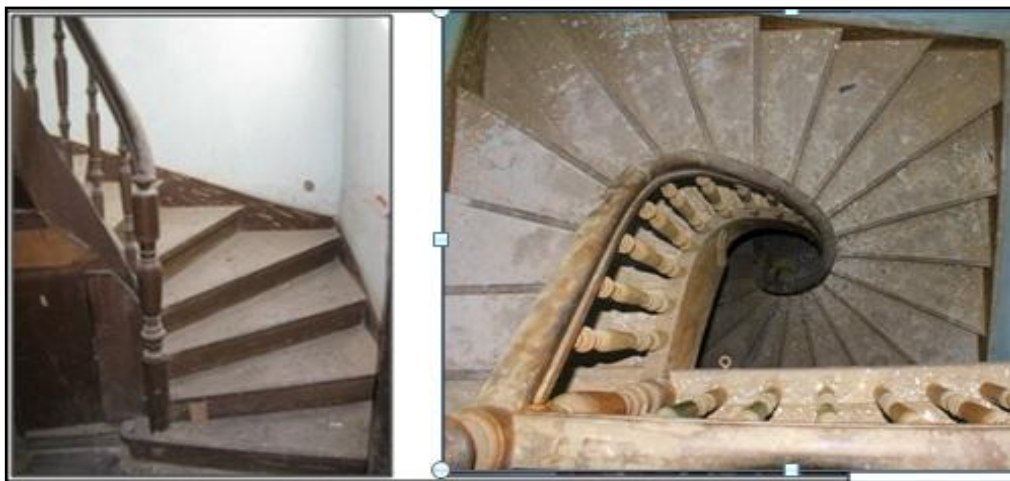
Figure 5.8 The building wooden staircase
