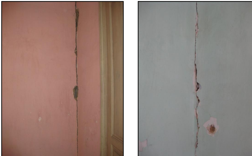
Figure 5.70: Wall separation along the interface between primary and secondary walls
