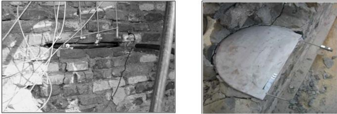
Figure 3.6 Placing the flat jack in the masonry wall and Relation between the contact area of the flat jack and the real area of the realized cut (Timchenko 2000).
