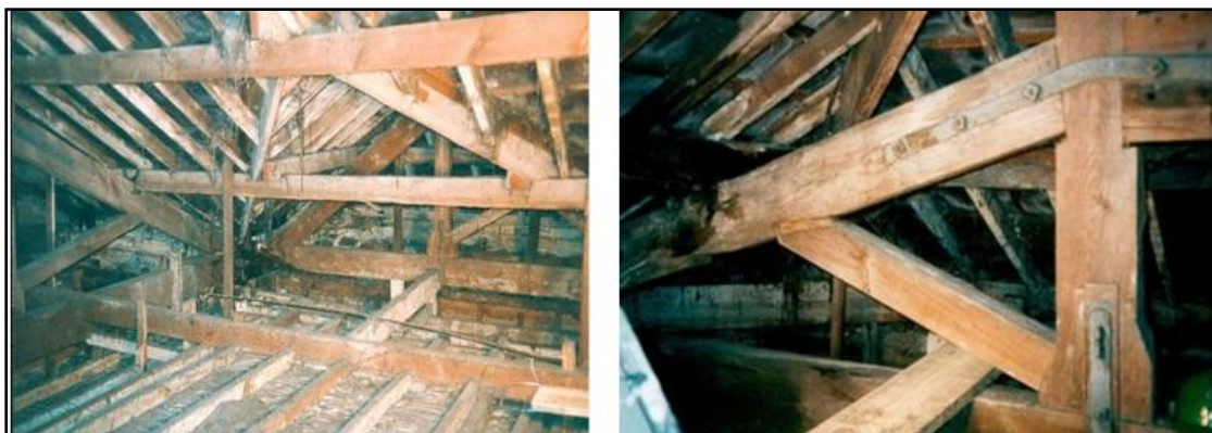
Figure 2.40 Decay aspects in roof timber
