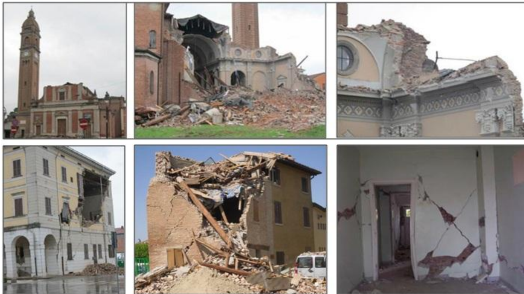
Figure 2.29 Out of plane failure in historic masonry buildings (Decanini L et al 2012, Parisi, F.; Augenti, N.2012, and Doğangün et al 2008)
