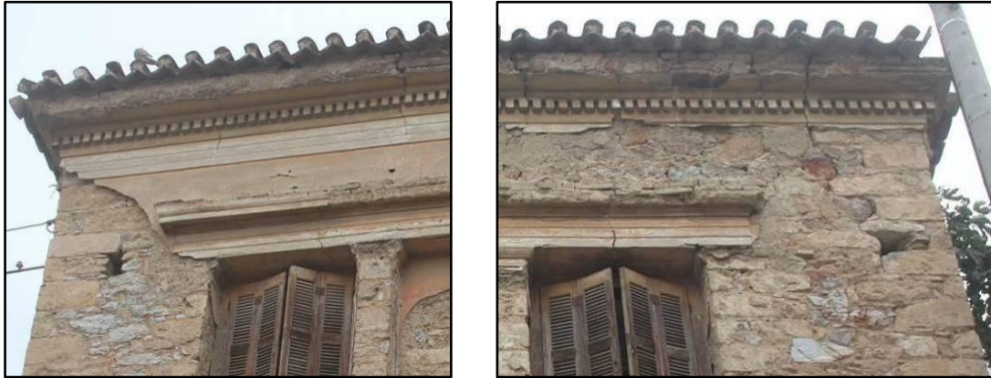
Figure 5.68: Cracking of the wall crowning
