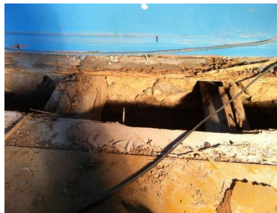
Figure 5.21: Wall recesses where the beams of ground level floor are supported
