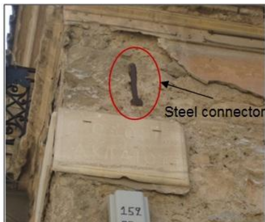
Figure 5.18: Steel connector tying orthogonal walls and roof
