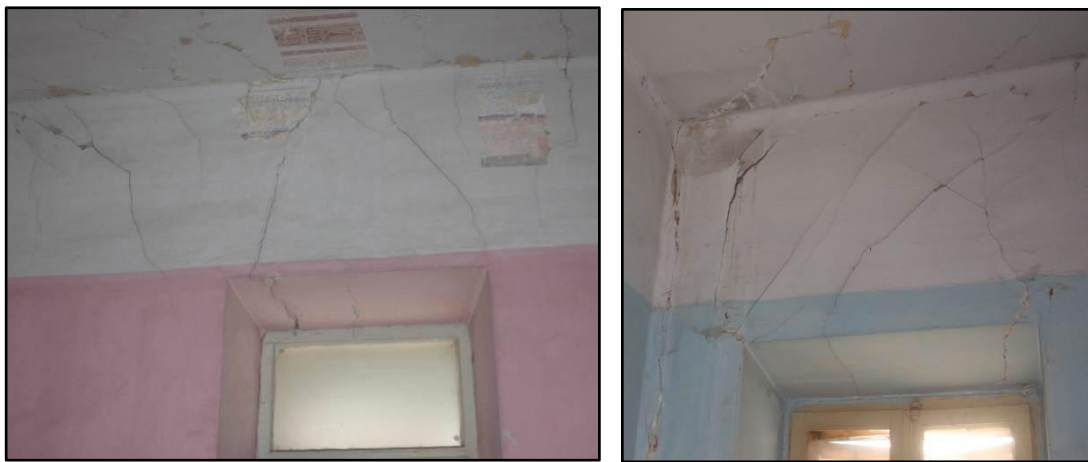
Figure 5.72: Masonry cracking of external wall above windows
