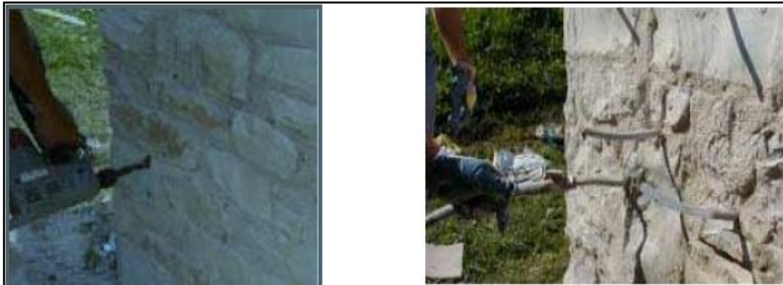
Figure 5.79: Process of drilling (left) and grouting (right)
