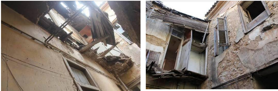
Figure 5.47: Collapsed galleries
