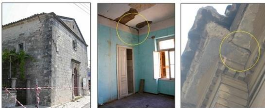
Figure 2.34 Cracks aspects in historic traditional masonry buildings in Greece (Abdelmegeed M. 2014)
