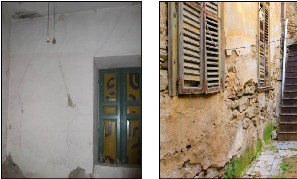
Figure 5.40: Wall cracking (W3-in, and W3-ex of ground floor)
