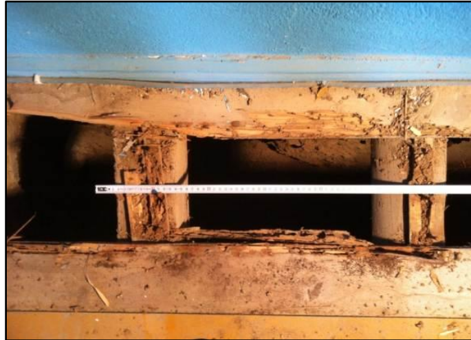
Figure 5.22: Spacing of beams of ground level floor
