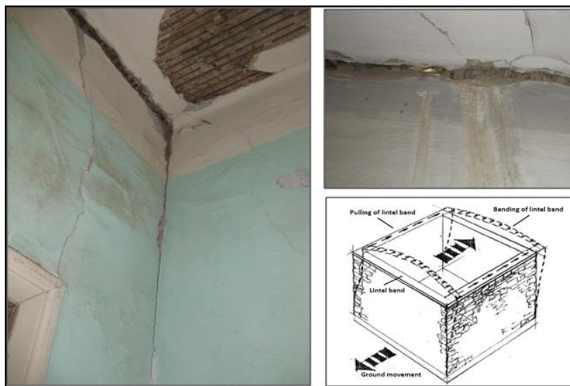
Figure 5.42 Horizontal cracks at the connection part between wall 3 and the roof in the 1 st floor
