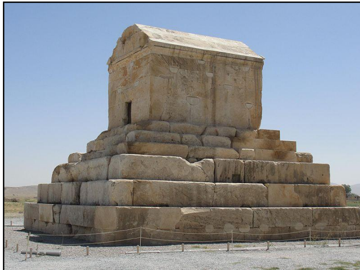
Figure 4.18 Tomb of Cyprus is said to be the oldest base isolated structure in the world (Wikipedia, 2014)
