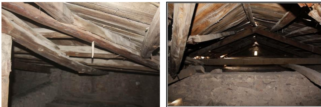
Figure 5.45: failure of truss member
