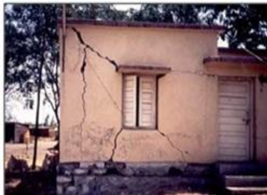
Figure 2.6 Typical wall cracking (Abdessemed 2003)
