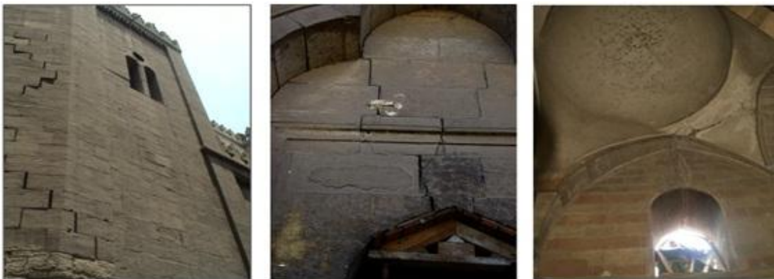
Figure 2.36 Cracks aspects in historic traditional masonry buildings in Egypt (Abdelmegeed M. 2010)
