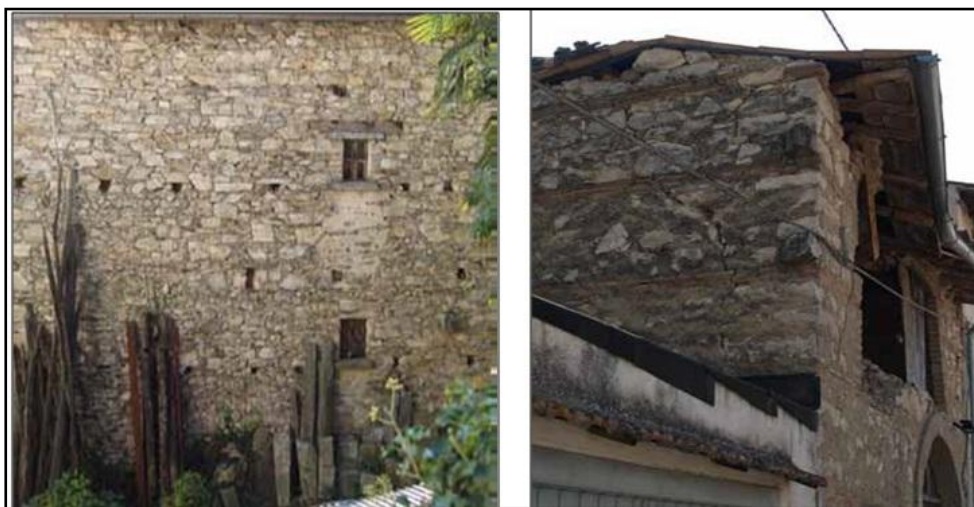
Figure 1.53 Un-coursed semi-dressed stone masonry walls (Bothara and Brzev 2011)
