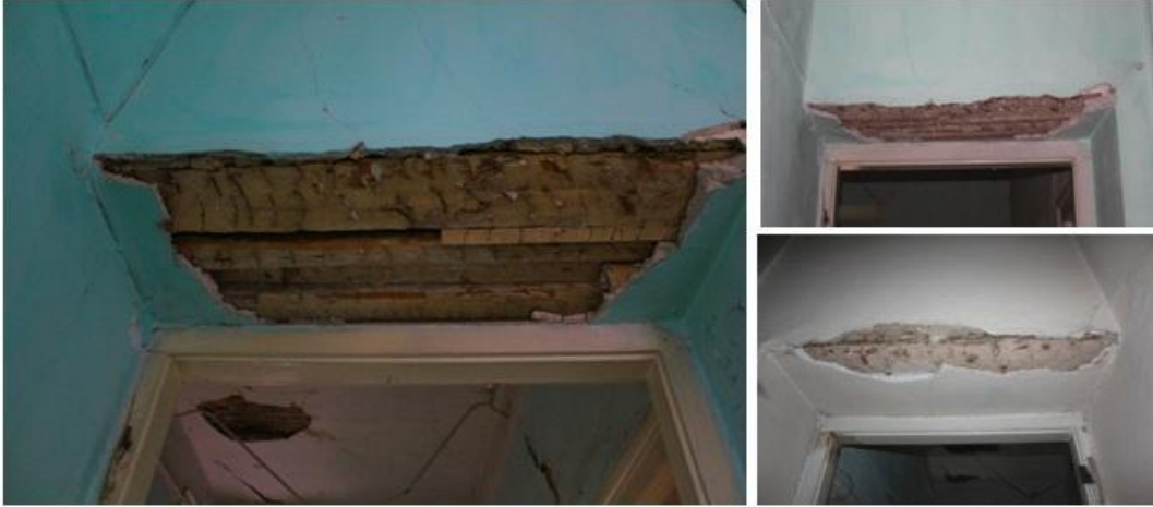
Figure 5.35: Typical lintel of internal opening
