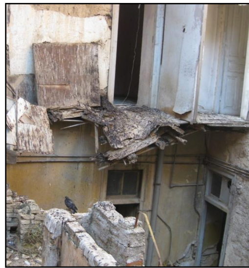
Figure 5.34: Typical gallery in a state of collapse.
