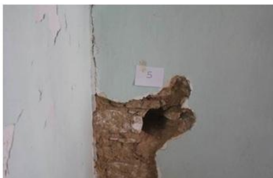
Figure 5.48: Removal of stone D7-MS
