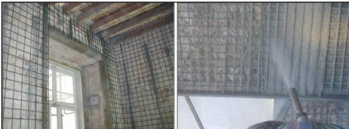
Figure 4.4 Masonry walls strengthening with steel mesh inside the building (Rashadul 2008).
