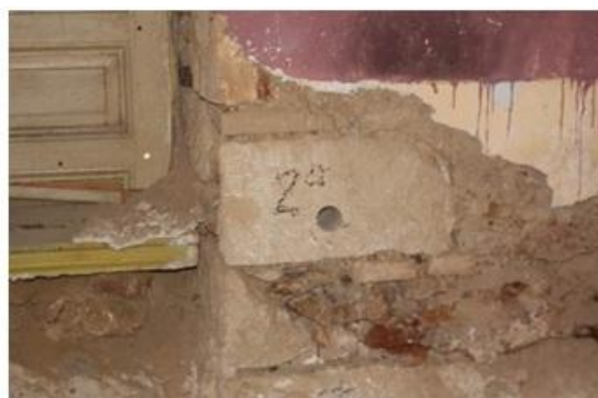
Figure 5.49: Drilling of core D10-LS
