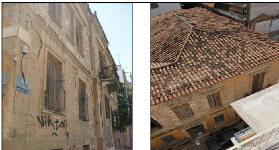
Figure 5.5: View of Aktaiou building house
