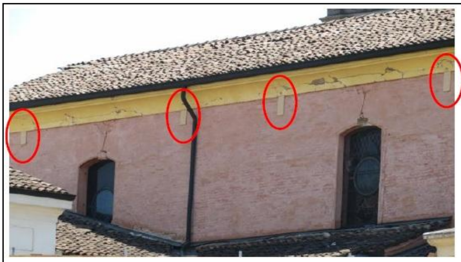
Figure 1.22 exterior views showing the tie timber element rods
