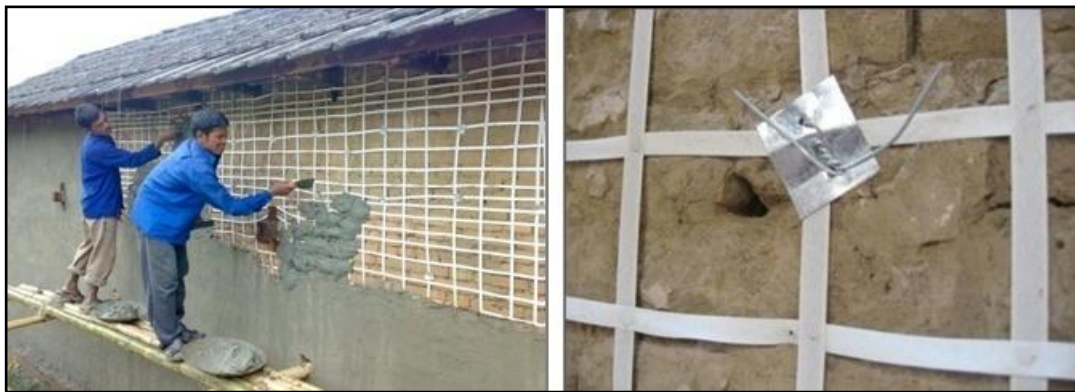
Figure 4.5 Implementation of PP band method of retrofitting and anchorage throughout the wall (Mayorka and Meguro 2008)
