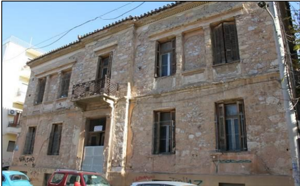
Figure 5.11: Aktaiou building facade (main façade) – Wall 1
