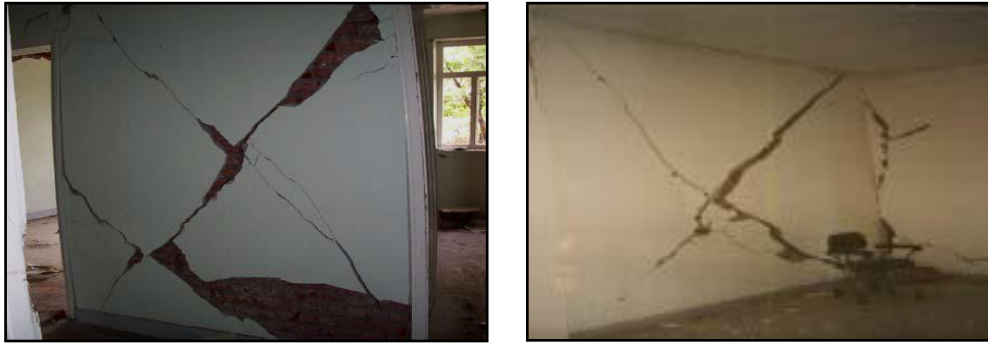
Figure 2.18 The form of double-diagonal shear cracks (Boen 2001)
