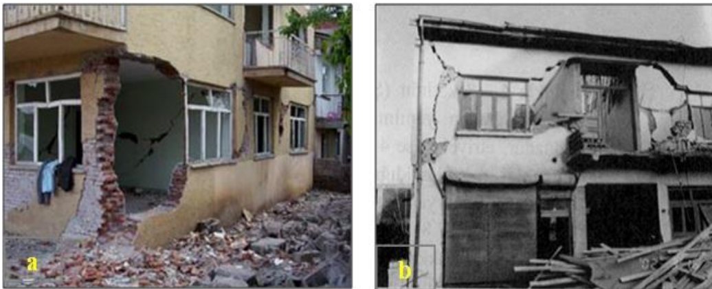
Figure 2.28- Collapse of a corner and vertical cracks near the corner for masonry buildings (Doğangün A. et al., 2008)
