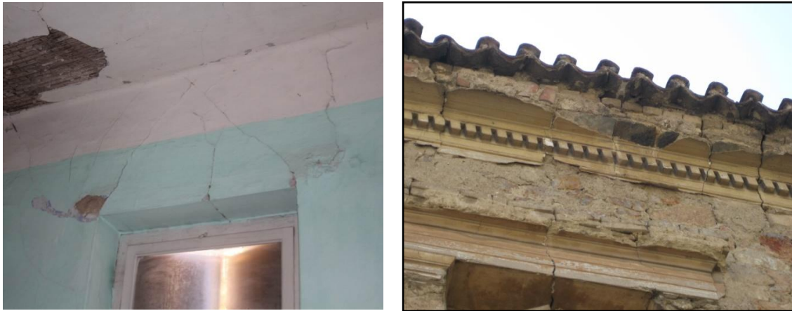
Figure 5.38: Lintel cracking (W1-in, 1 st floor) and vertical cracking at both the top (W1-ex, 1 st floor) of the building
