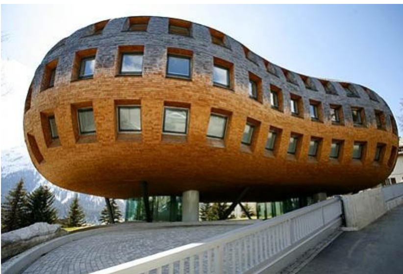
Figure 17. Chesa Futura St. Moritz 2000-2004 Foster and Partners
