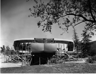
BASIC PLAN has four 18'-square wings and a central 18'-square core, giving 1,200 square feet of living space, plus basement. Bathrooms, closets and bedrooms are grouped in core. Plastic wings are placed at ends for space of entry, so that two-headed living, work or study area of any type, can be used.
