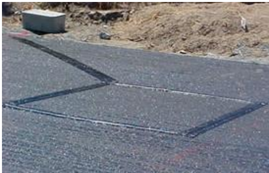
Figure 4-5: Simple loop detector.
