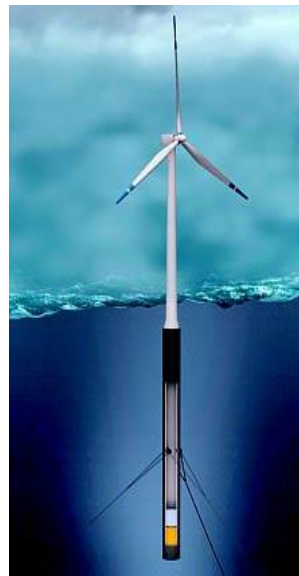
Figure 4.2: Description of the spar buoy floater of the OC3
