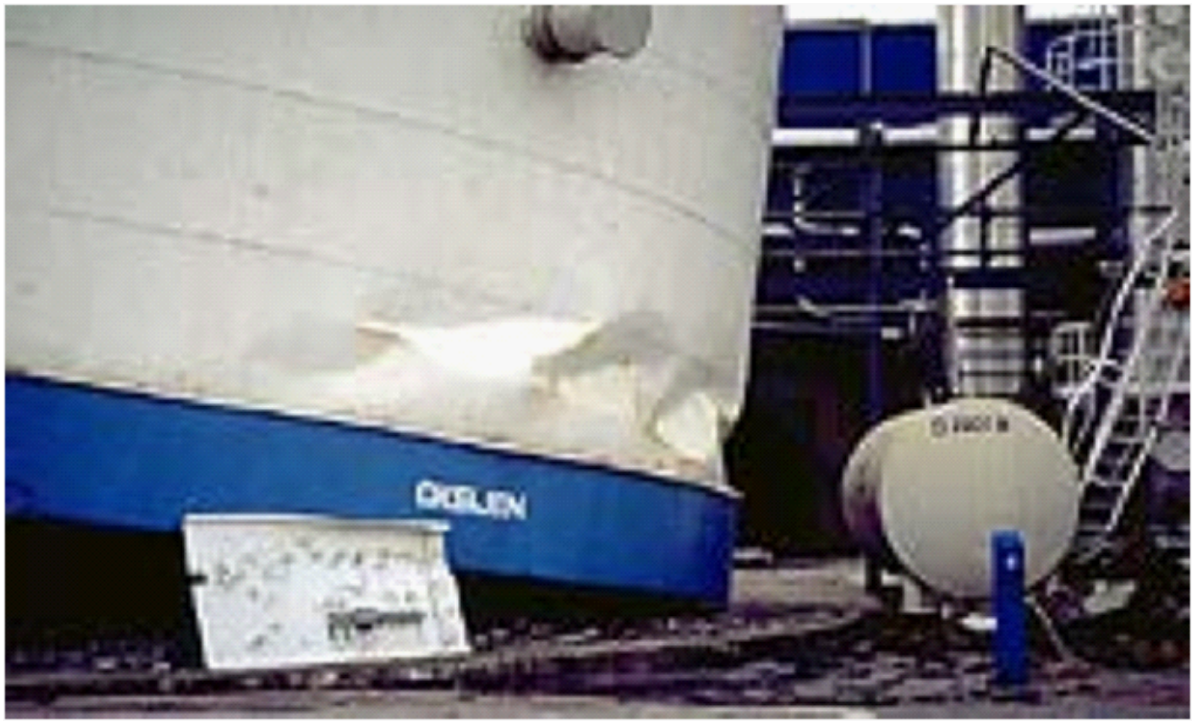
Figure 13: Buckling of the outer stainless steel shell in liquid oxygen tank ( http://nisee.berkeley.edu/turkey/Fturkch4.pdf )
