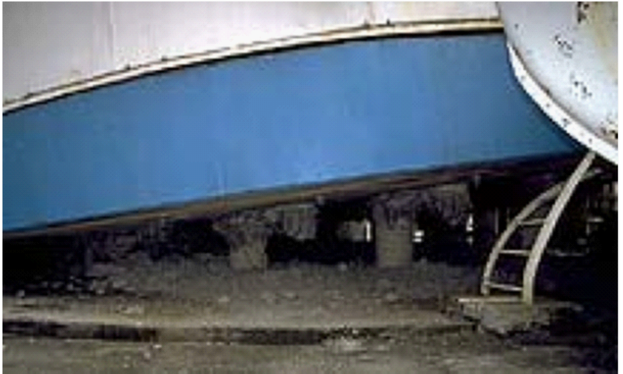
Figure 14: Failed columns beneath slab under liquid oxygen tank, Habas facility ( http://nisee.berkeley.edu/turkey/Fturkch4.pdf )
