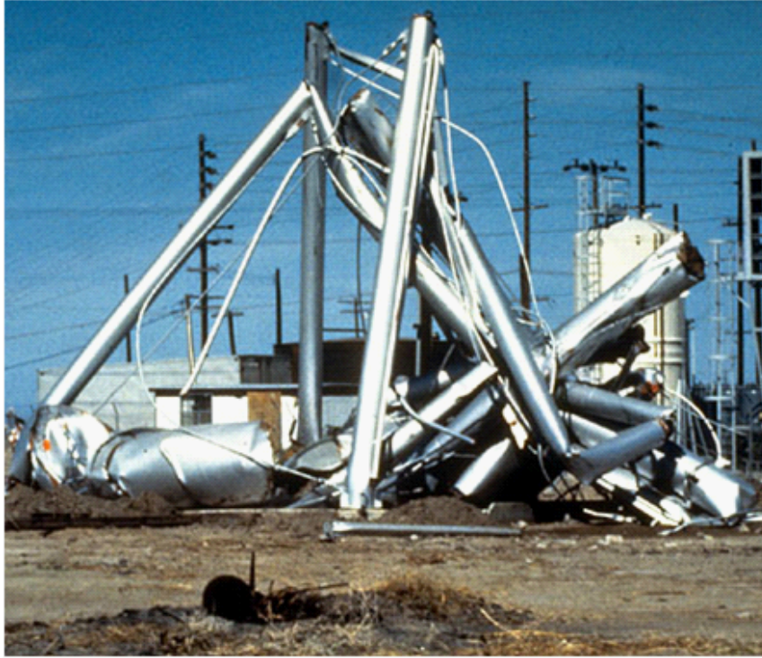
Figure 7: Collapse of a steel tank during the 1979 Imperial Valley Earthquake. ( http://nisee.berkeley.edu/jpg/6257_3021_0662/IMG0037.jpg , Steinbrugge Collection, Earthquake Engineering Research Center, UC Berkeley )
