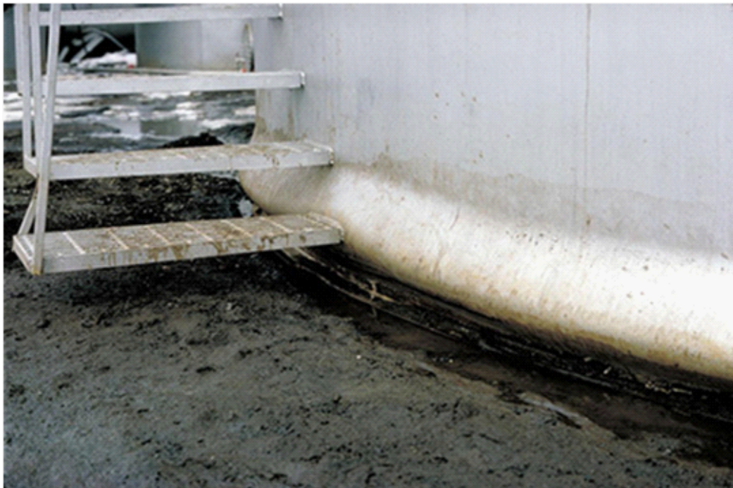
Figure 3: Tank with “elephant’s foot” buckle at the base in the 1964 Anchorage, Alaska earthquake ( http://www.fema.gov/earthquake/fema-e-74-reducing-risks-nonstructural-earthquake-damage-31 , PEER, Steinbrugge Collection, No. S2508)
