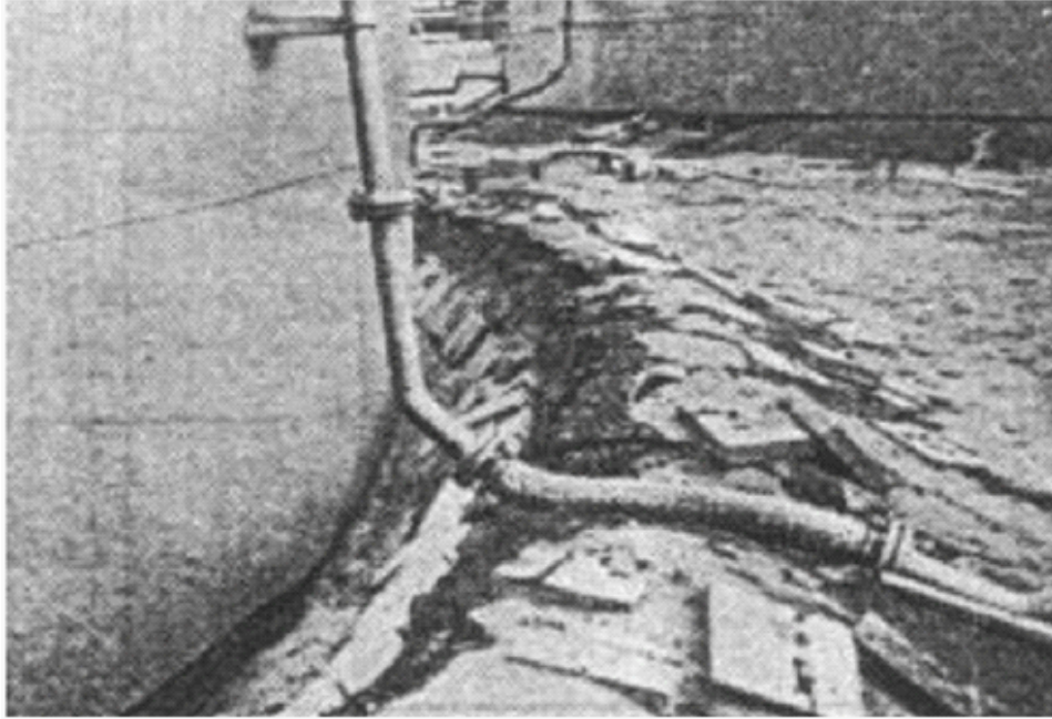
Figure 5: Settlement of tank on unimproved ground (Watanabe 1966)
