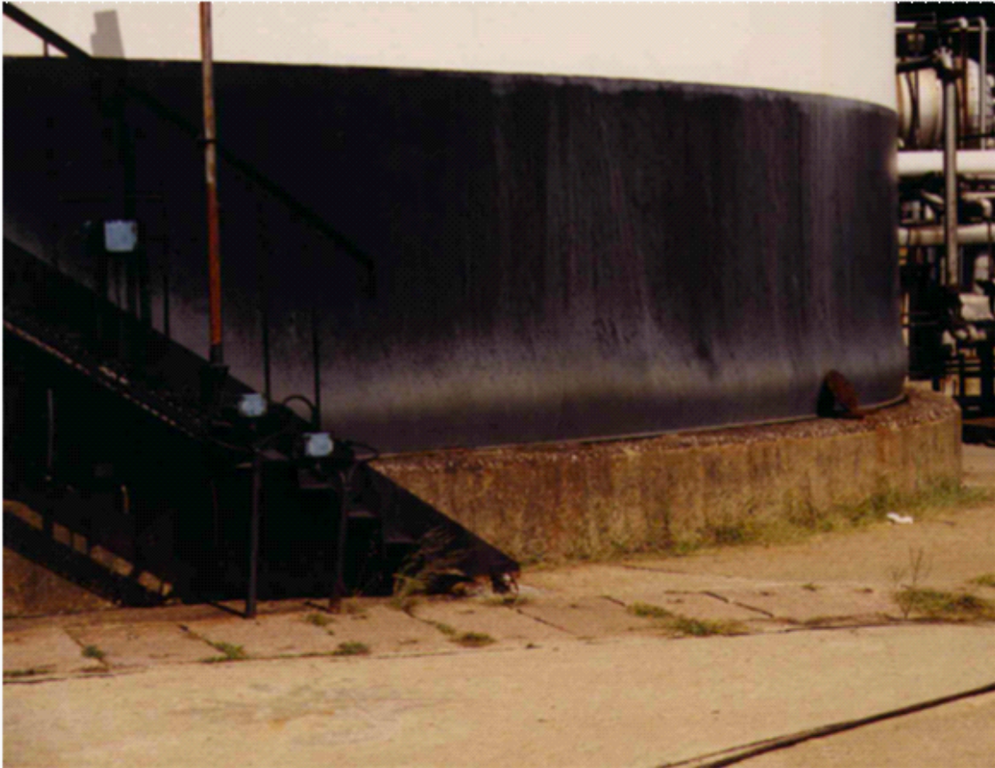
Figure 17: Elephant-foot bulge (Hosseinzadeh (2008))
