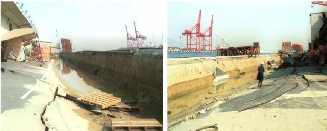
Figure 1.3 : Large settlement of embankments behind quay walls at Kobe, Japan 1995 earthquake
