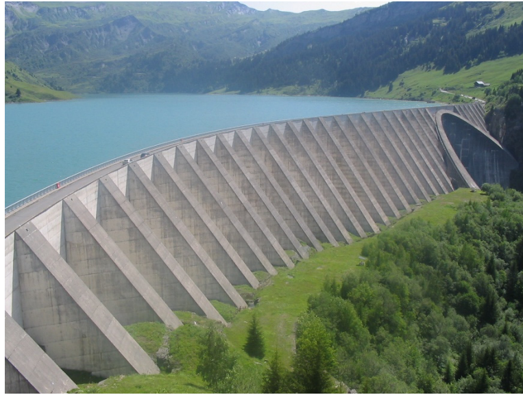
Figure 3.18. A reinforced concrete water dam analyzed with Non-Classical Damping. Water's Damping Ratio is negligible compared with Dam's.
