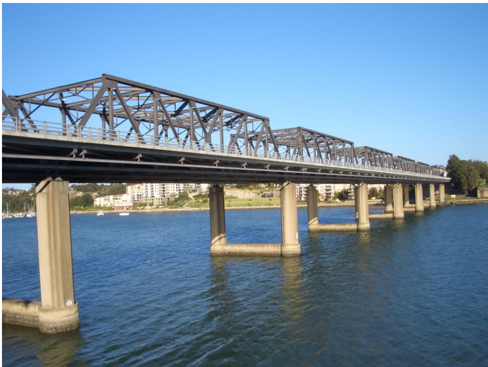
Σχήμα 1 - 2 : Fourth Rail Bridge, Edinbrugh Scotland (πάνω), Iron Cove Bridge, Sydney Australia (κάτω)
