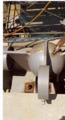
Joints of the ring truss.
