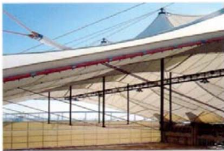
Suspension cables running through the roof.
