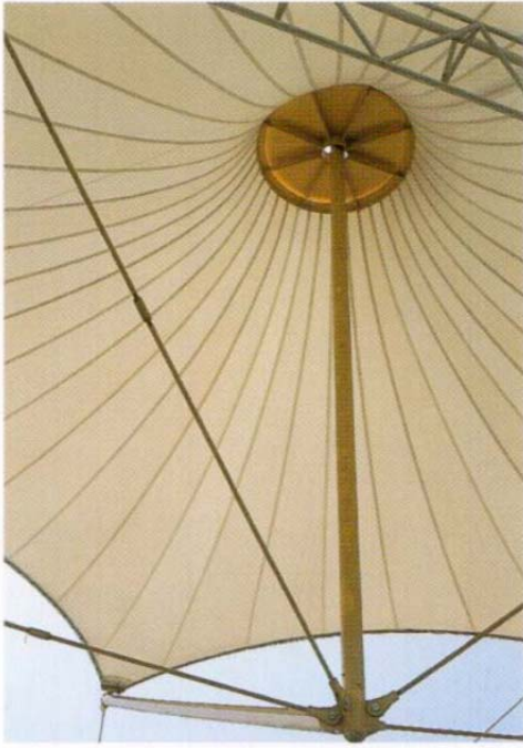
Upward view of the membrane roof.
