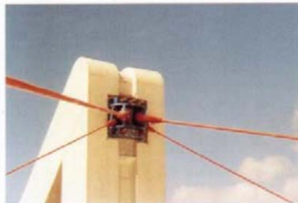
Anchor block for the suspension cables.
