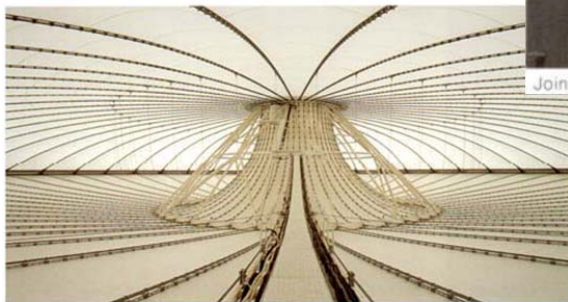
Interior of the air-inflated membrane with the hybrid structure.
