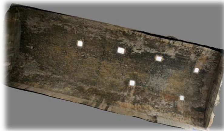
Figure 3.10 3D textured model of the interior roof of the Temple of Hephaestus. In this case the roof
