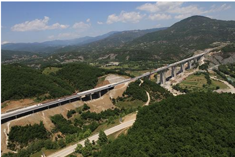
Figure 25: Arahthos-Peristeri Bridge in Egnatia Highway
