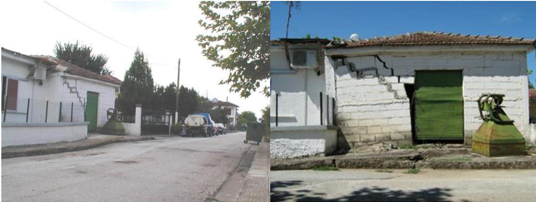
*Figure 5: Damages due to land subsidence in West Thessaly basin. The cracks in the stonework on the left photo by Apostolidis and Georgiou (2007) evolve, despite the repairs even eight years after, as seen in the right photo taken by the author in 2015.*
