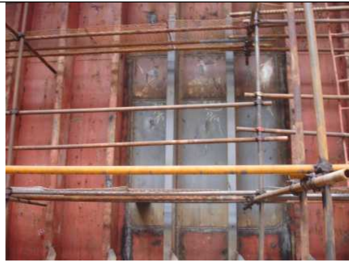
REPAIRS UNDER PROGRESS
