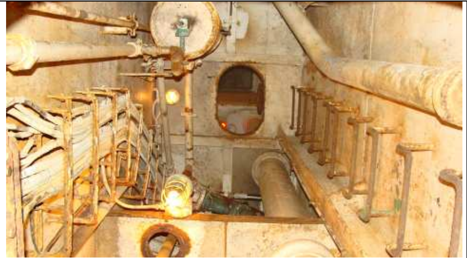
ENTRANCE TO BOW THRUSTER ROOM
