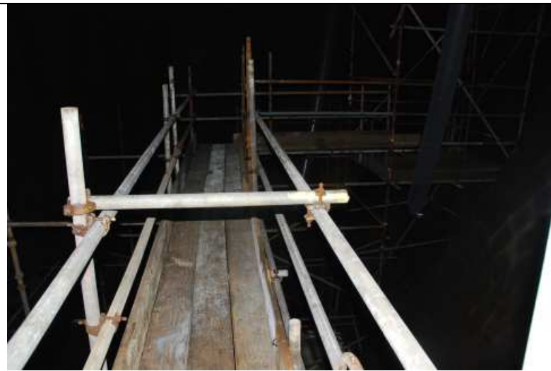
EXAMINATION WITH SCAFFOLDING
