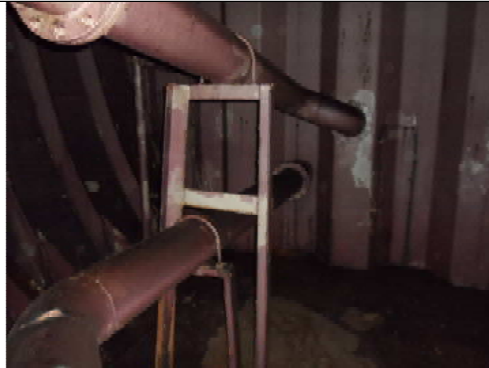
TANK AT SIDE
