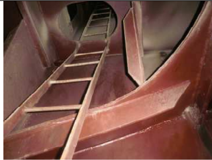
COFFERDAM IN PUMP ROOM
