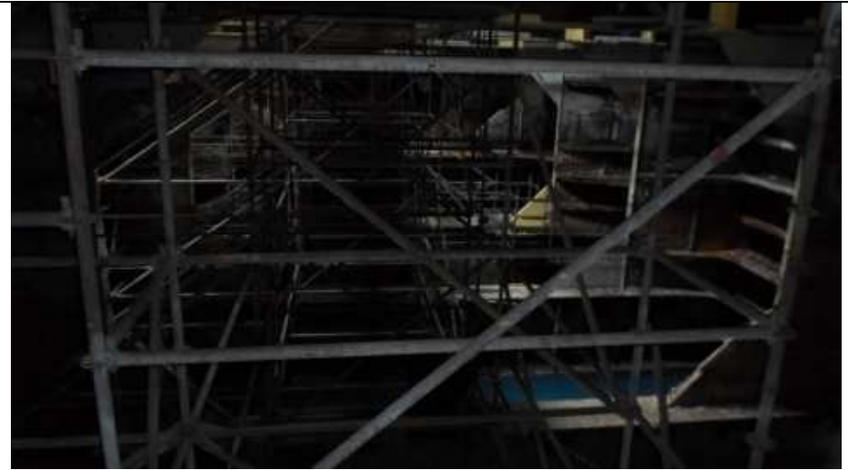
EXAMINATION WITH SCAFFOLDING
