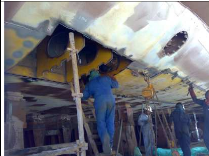
REPAIRS UNDER PROGRESS
