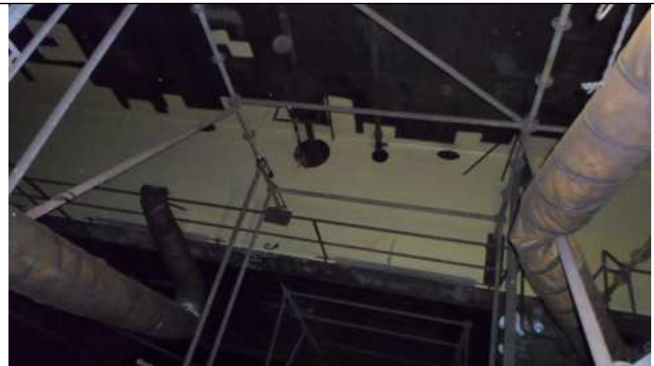
EXAMINATION WITH SCAFFOLDING
