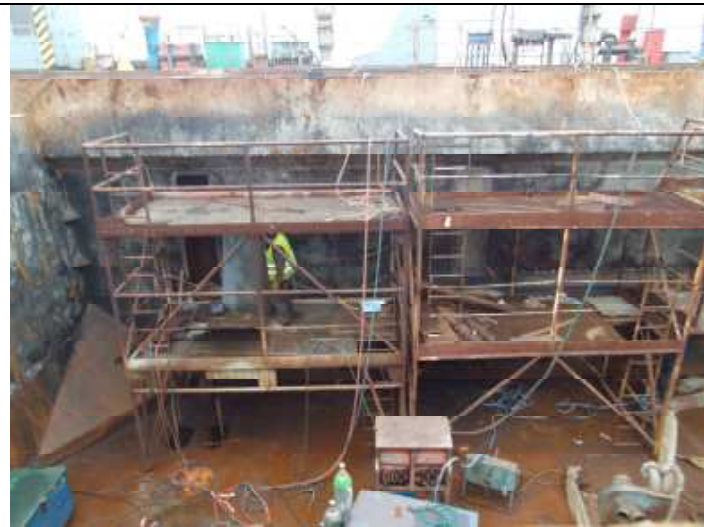
REPAIRS UNDER PROGRESS
