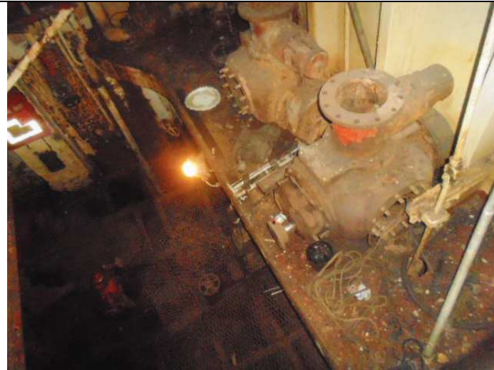
GENERAL VIEW DURING OVERHAUL
