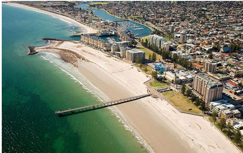
Fig. 1.2. Erosion down-drift of a coastal defense system in a beach with undue human pressure in Glenelg, Adelaide, Australia (photo: Web-Based Geohazards Project, University of Adelaide, www.coastalerosionsa.wordpress.com ).
