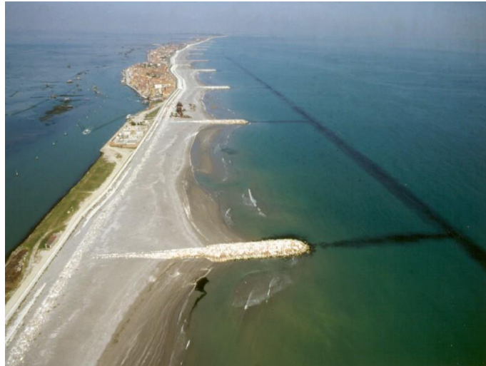
Fig. 5.3. View of a composite coastal protection project including submerged breakwaters in Pellestrina island in Venice, Italy (photo: DELOS project, www.delos.unibo.it ).
