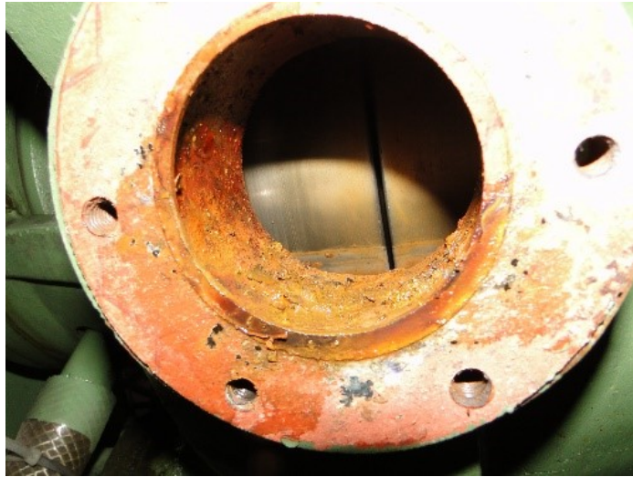
Figure -4: WB water outlet opened for inspection.
