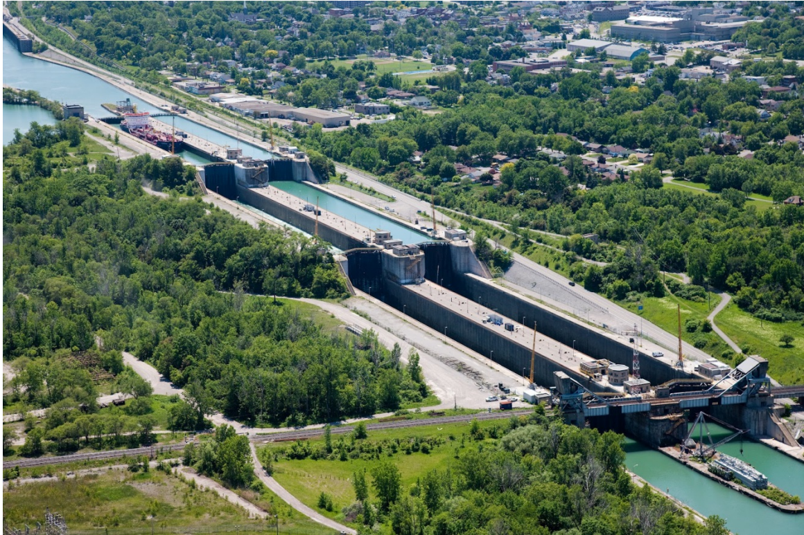
Figure 10 Welland Canal (Canada)
