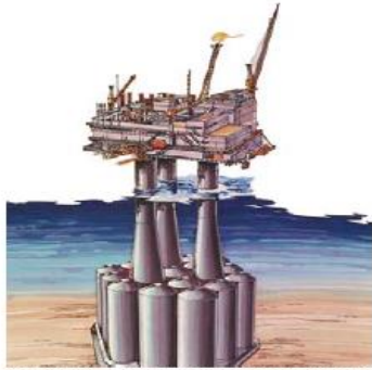
Figure 2.1: A typical Condeep design
