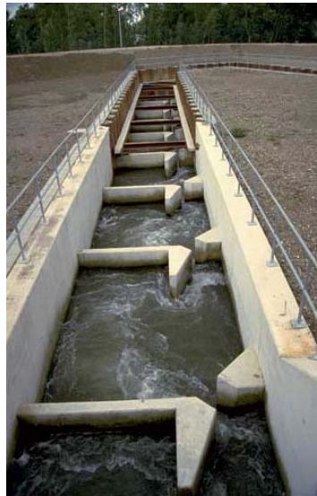
Figure 7.2 - 1: Vertical slot Fish-Pass, [source: (FAO, 2001)]
