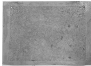
The cleaned surface
