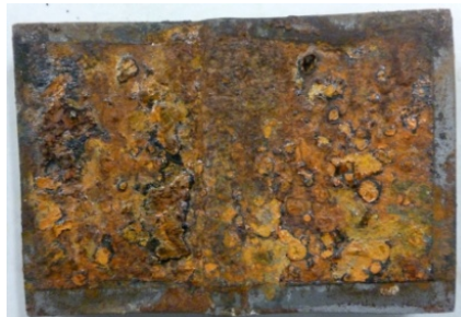
The corroded surface
