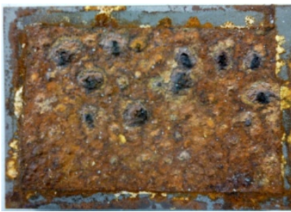
The corroded surface
