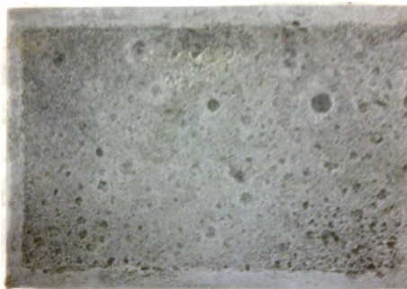
The cleaned surface
