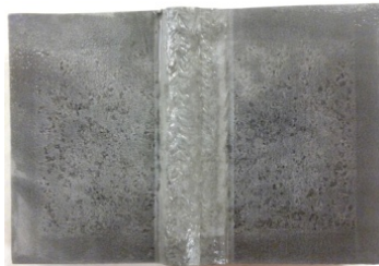
The cleaned surface
