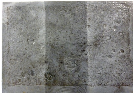
The cleaned surface
