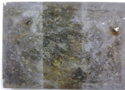
The cleaned surface
