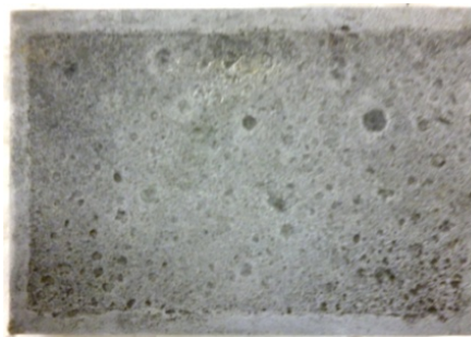
The cleaned surface
