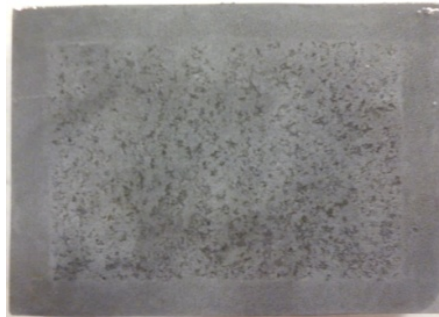
The cleaned surface
