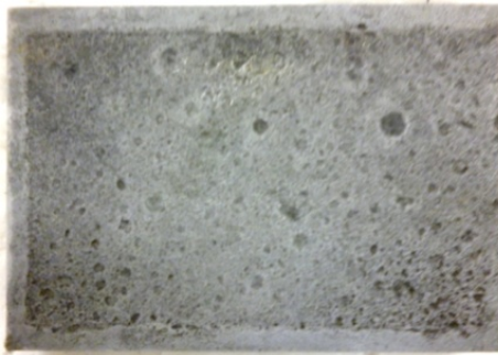
The cleaned surface
