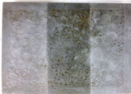
The cleaned surface
