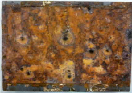
The corroded surface
