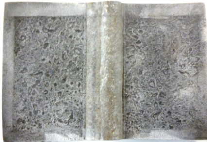
The cleaned surface
