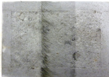
The cleaned surface
