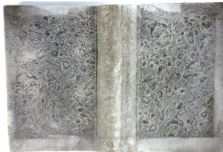
The cleaned surface
