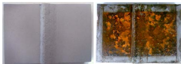
The sandblasted surface
