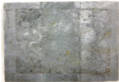
The cleaned surface
