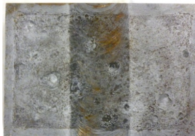
The cleaned surface
