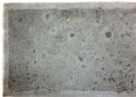
The cleaned surface
