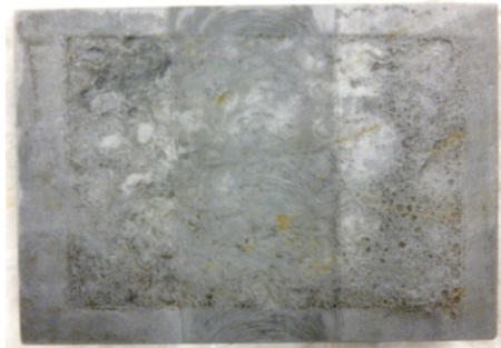
The cleaned surface
