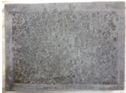
The cleaned surface
