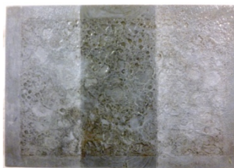
The cleaned surface
