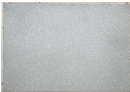
The sandblasted surface
