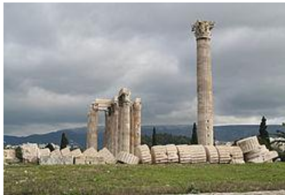
Figure 2: Overturning of a free-standing pillar after an earthquake.
