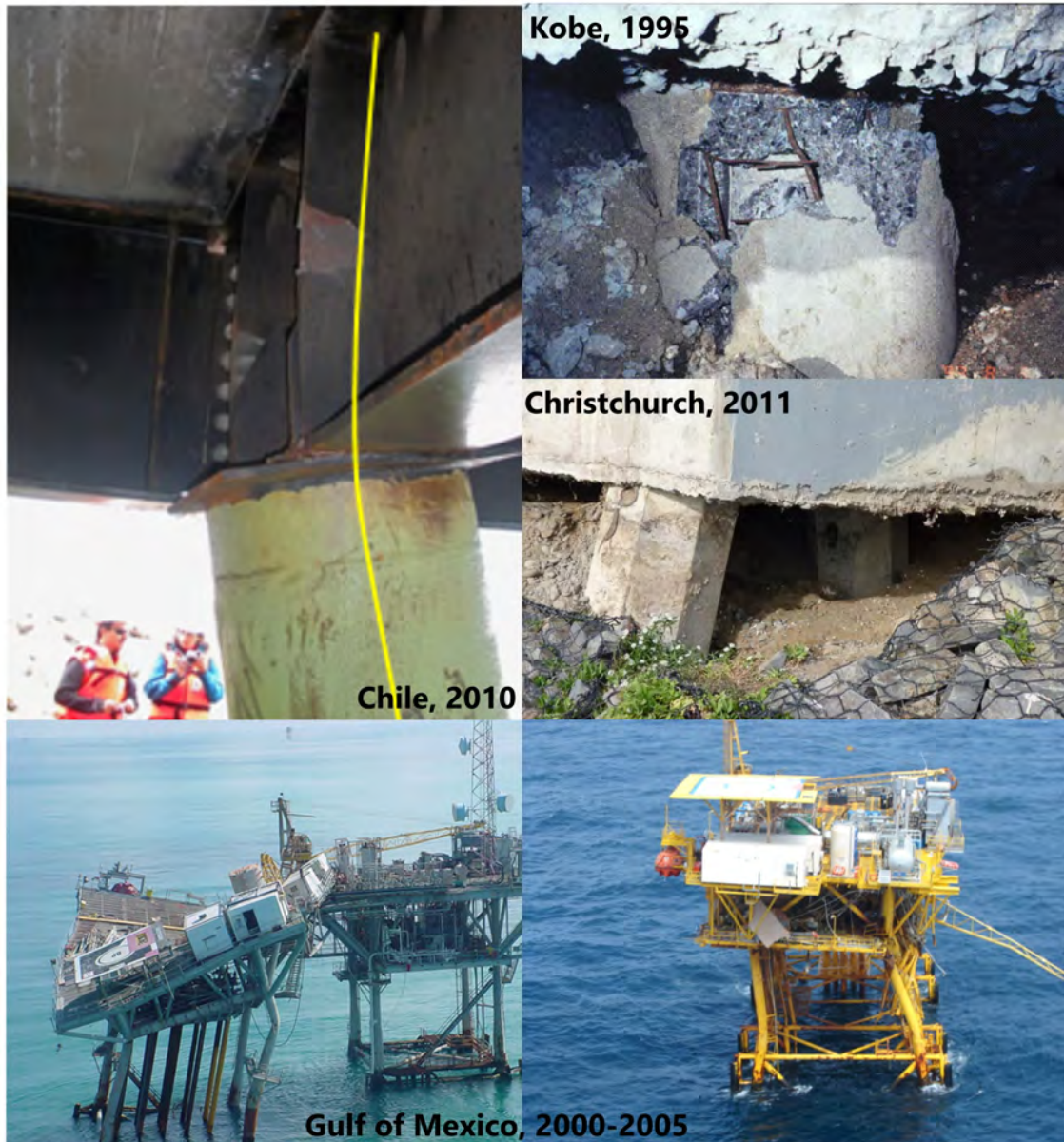
Figure 1.1: Indicative failures of laterally loaded piles around the world.
