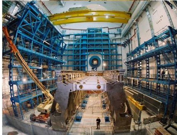
Figure 4.2: The ATLAS cavern [25] with dimensions 35 x 55 x 40 m [58]
