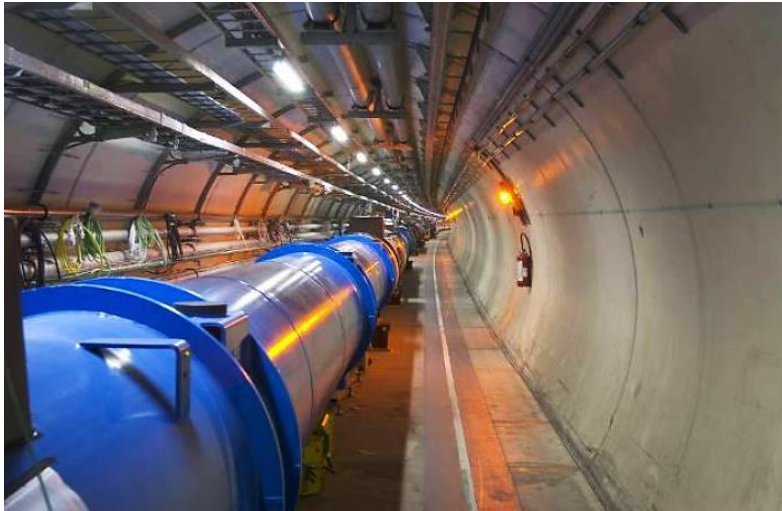
Figure 3.1: The LHC tunnel [21]
