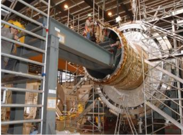
Figure 4.24: The cylindrical solenoid magnet enters the surface of the LAr Calorimeter [21]
