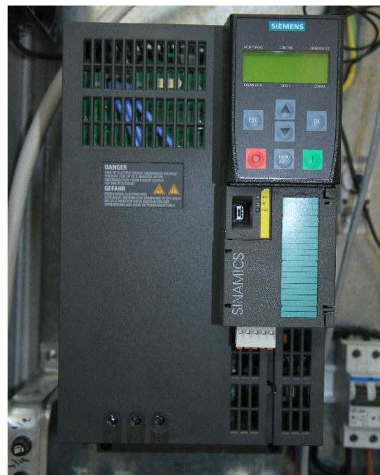
Figure 45 – Regenerative inverter.
