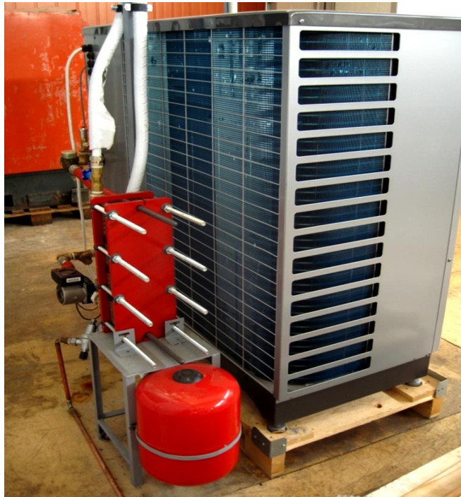
Figure 34 – Rear side view of the installed commercial heat pump before its retrofitting with the expander prototype. The closed water circuit and its heat exchanger can also be seen as well as the fins of the air/refrigerant evaporator heat exchanger can be clearly seen.
