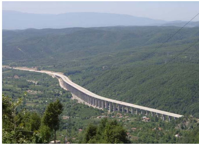
Figure 14: Bolu Viaduct, Turkey
