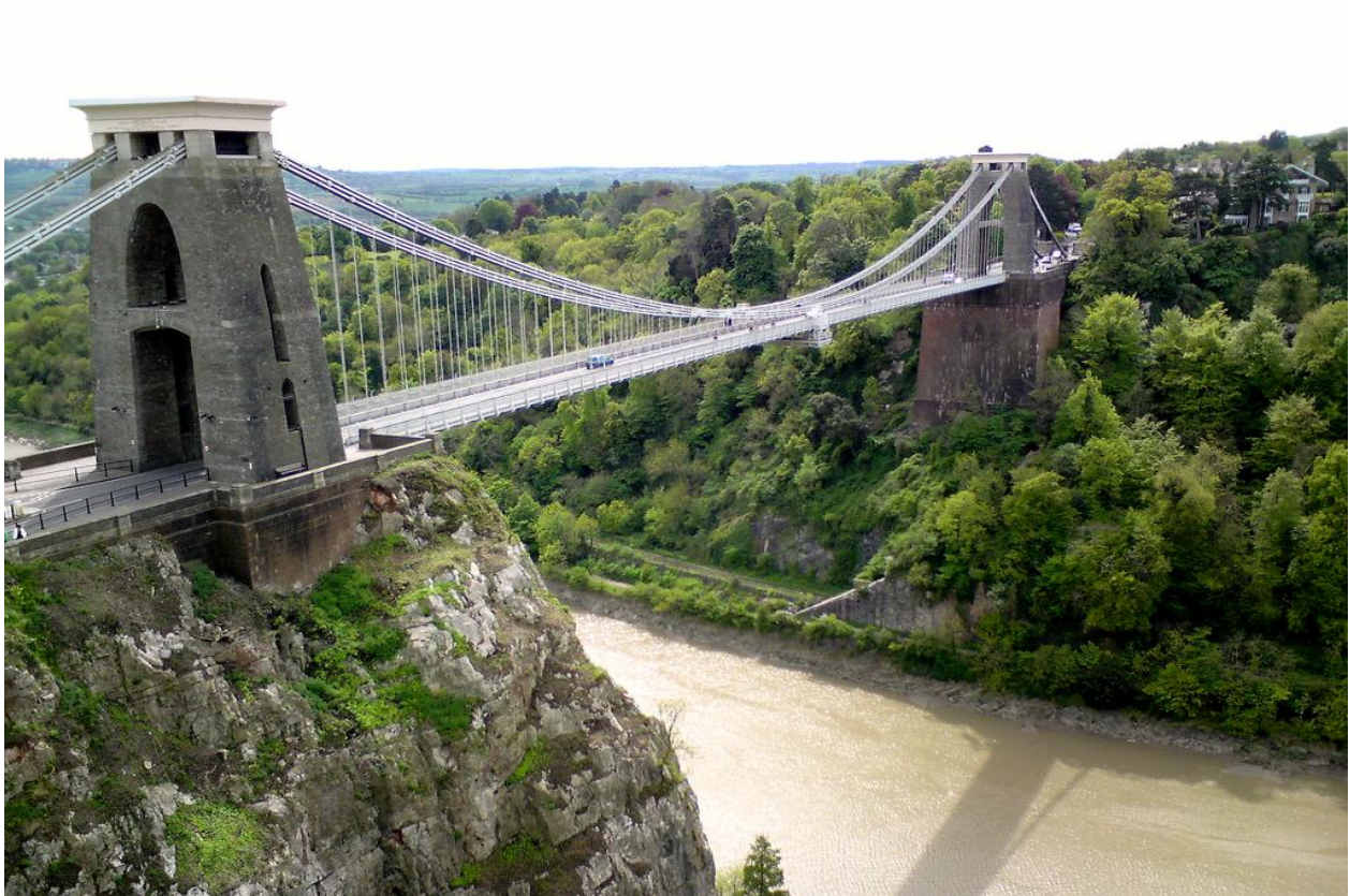
Σχήμα 1.1: Clifton Bridge (Briston, England 1864)
