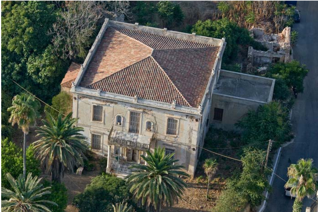
Image 6.1 A typical aerial photograph of the building in its present form
