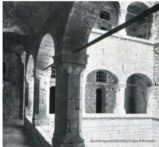
Image 1.5 Tie rods in Stonemasonry
