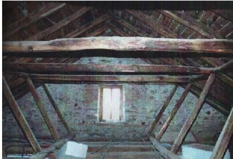
Image 1.3 Wooden Roof of Stone Structure
