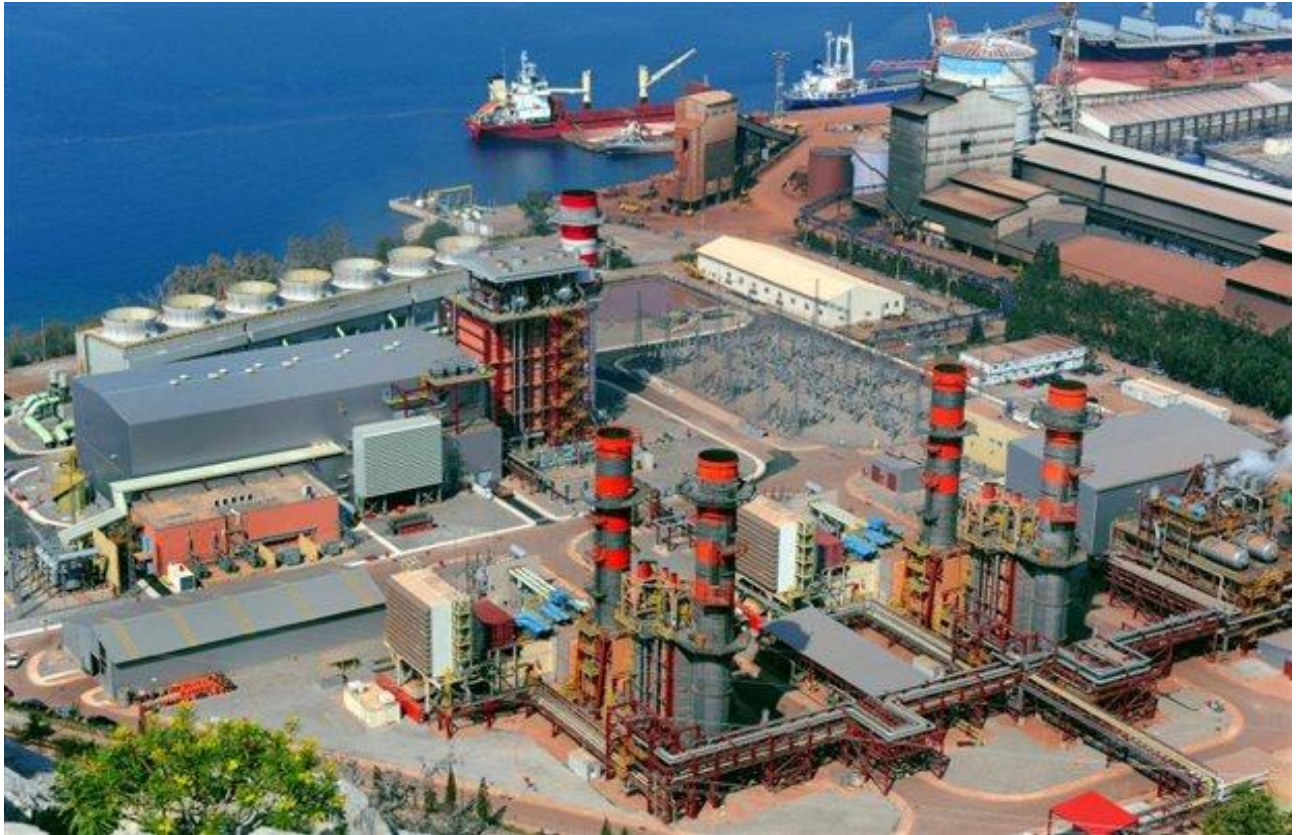
Figure 8: Cogen Power Plant beside the Aluminum of Greece Plant
