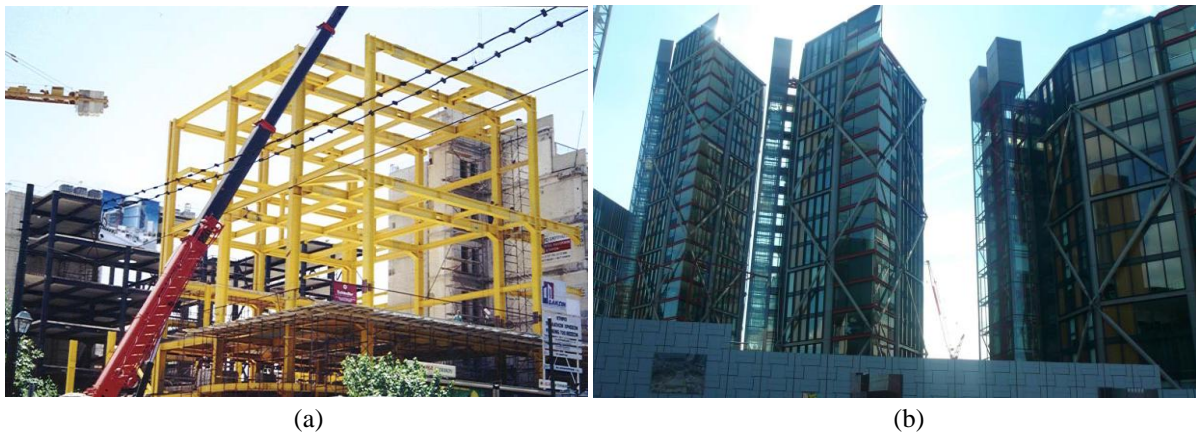
Figure 1.2: (a) Moment-resisting frames (b) Concentrically braced frames
