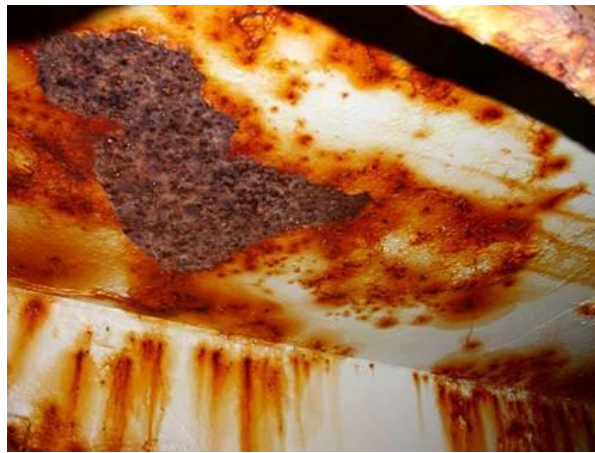
Figure 9: A ship's hull affected with rust. Extensive corrosion deteriorates the metal structure and can cause strength issues.
