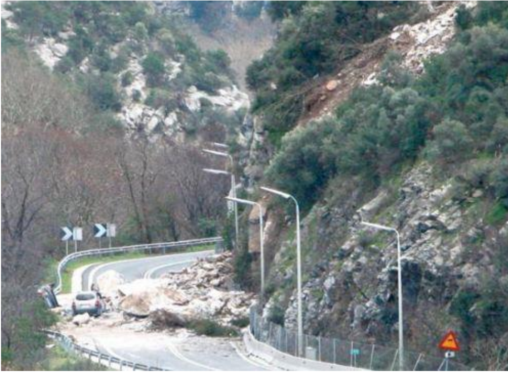
Figure 3.14: Rockfall at Tempe in central Greece
