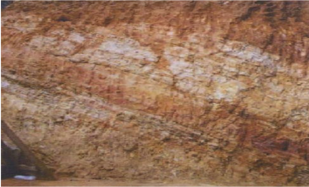
Figure 3.2: Residual soil derived from gneiss, exhibiting different zones inherited from the parent rock, representing heterogeneity, anisotropy and planes of weakness along the structure (Ortigao & Sayao 2004)
